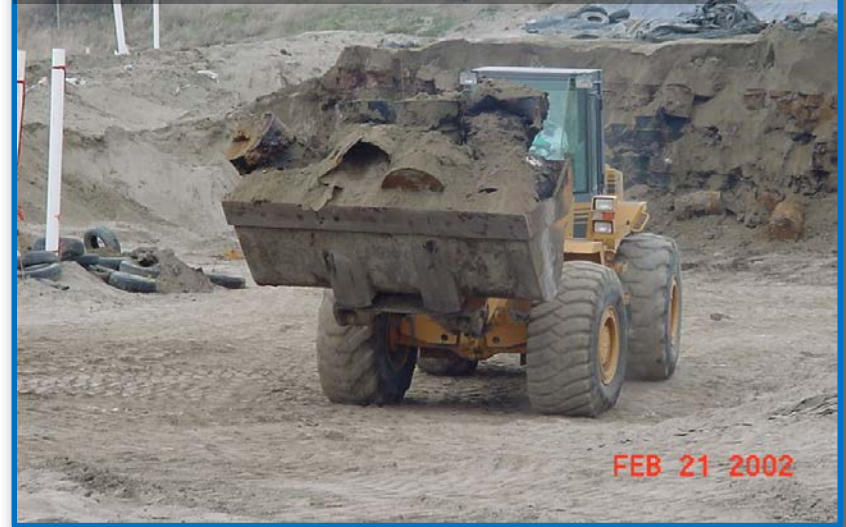
Zone B drum removal – 2002
