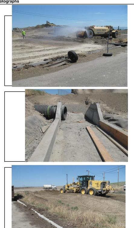
Photo # IMG-2992 **Brief Description** watering/compacting fill over 10" HDPE storm drain east of Compost area
