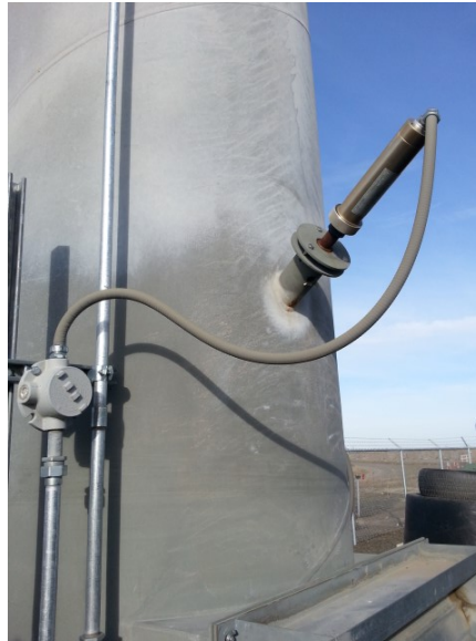
Coen Flame Scanner Assembly
