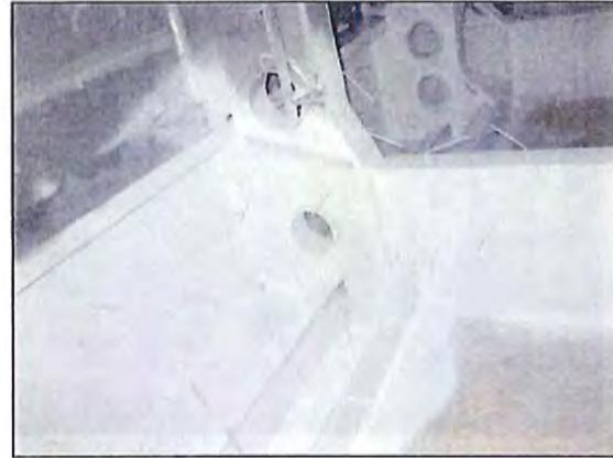
**The two burn pictures directly below are the surfaces there were welded for a pipe hanger. The coating was applied prior to the fix and the weld. This shows that the coating can tolerate repairs with minimal degradation of the coating in the area adjacent to the weld.**
