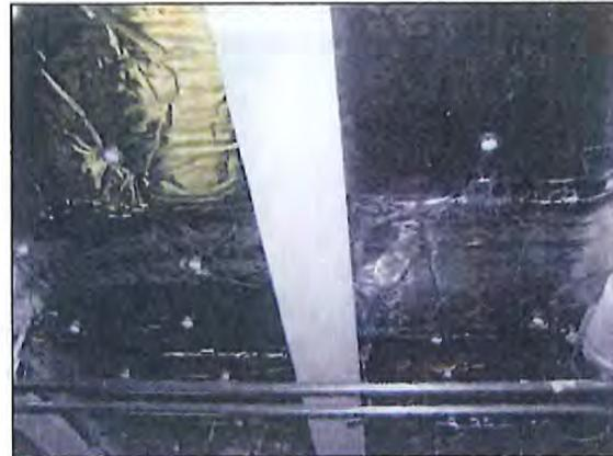
Delta T Marine applied to the outside wall of the vessel and framing supports to combat condensation/sweating. The coating is normally applied to 40-80 mils (1.0-2.0 mm) in a series of coats. By applying the coating to the side walls, stiffeners, overheads and shells of the vessel, protection is given as well as reducing radiant heat gain.
