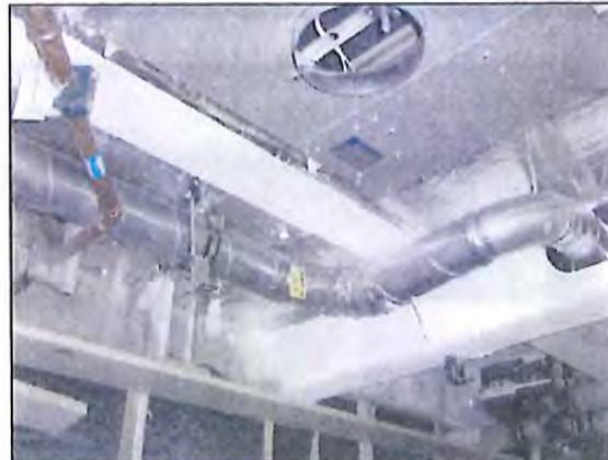
More applications using the coating in conjunction with conventional sound damping insulation. This method allows for thermal and sound control inside state of the art yachts. The pins and hangers also are used for structural fire protection.
