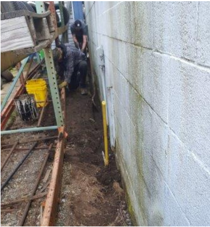
Digging Out Southern Drainage Trench
