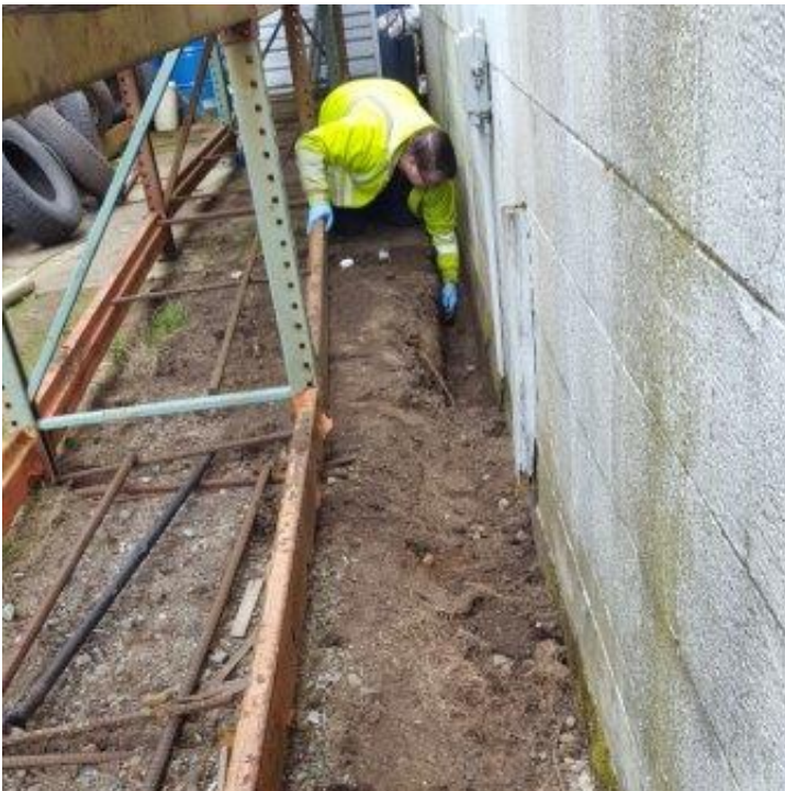
Sampling Southern Drainage Trench
