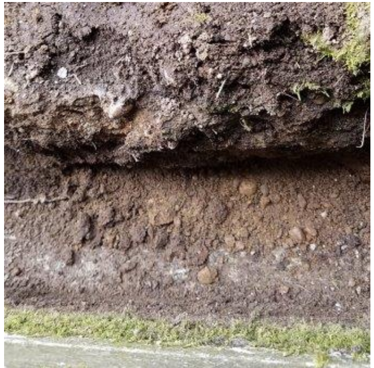
Close-up of Base of Footing Abutting Concrete Slab
