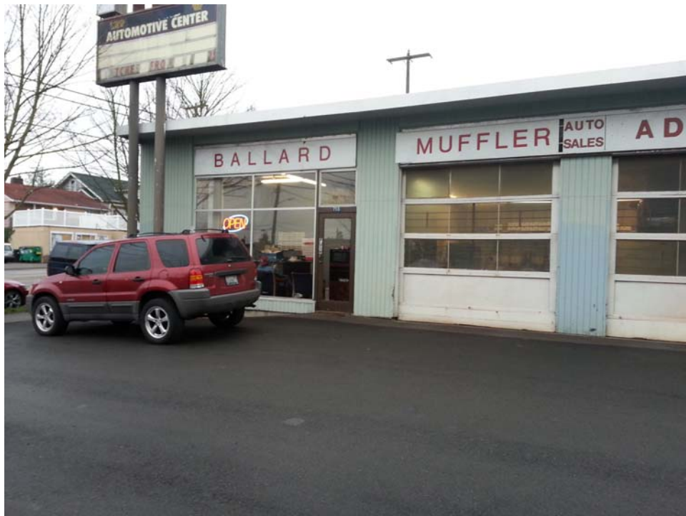
3.) View of the front of the Muffler shop at 7530 15 th Avenue NW.
