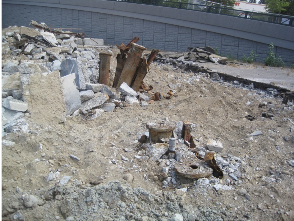
Photo 3: August 5, 2015. View of two of the dual-piston hydraulic lifts that were discovered and removed from the DOB site.
