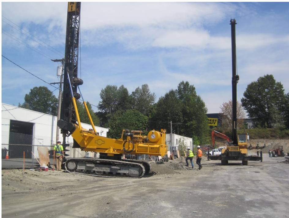
Photo 2: August 10, 2015. Large diameter borings for soldier piles were installed on 10-foot centers along the north side of the Property adjoining the former Bellevue Lincoln Mercury site. No evidence of potential contamination was identified during the drilling. Soldier piles were also installed along the east and south edges of the Property.
