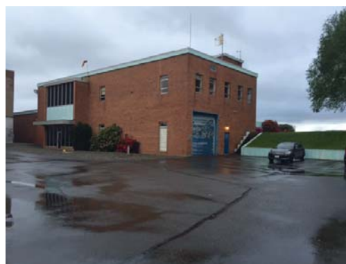
Filtration Basin view to north
