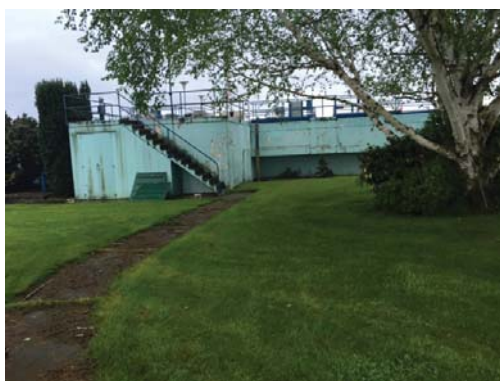
Sedimentation Basin north side
