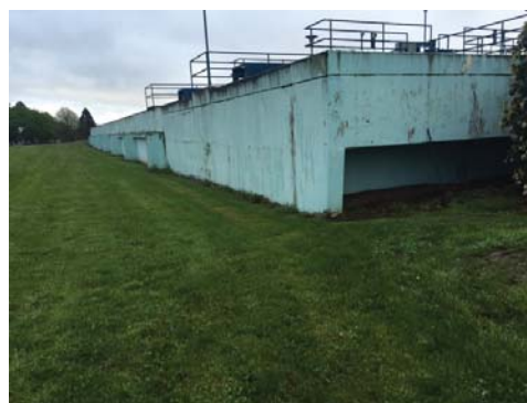
Sedimentation Basin east side
