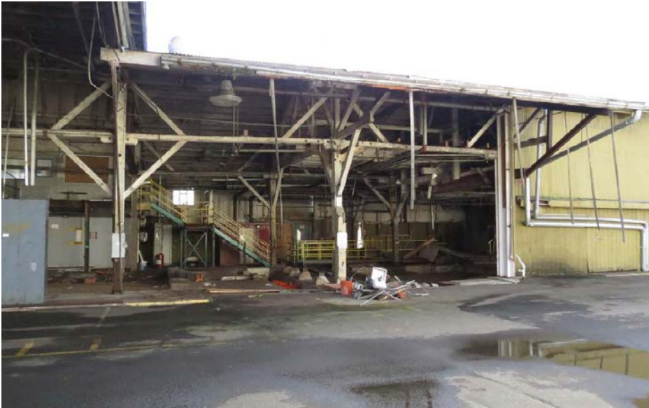
Seaport Landing - Planer Mill - Building 8.3
