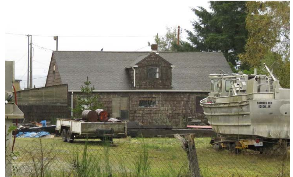
Pakonen Boatyard - House - Building 15
