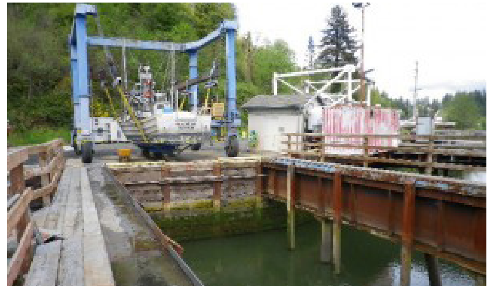
Boatyard lift and assembly docks at the Port of Toledo, OR.
