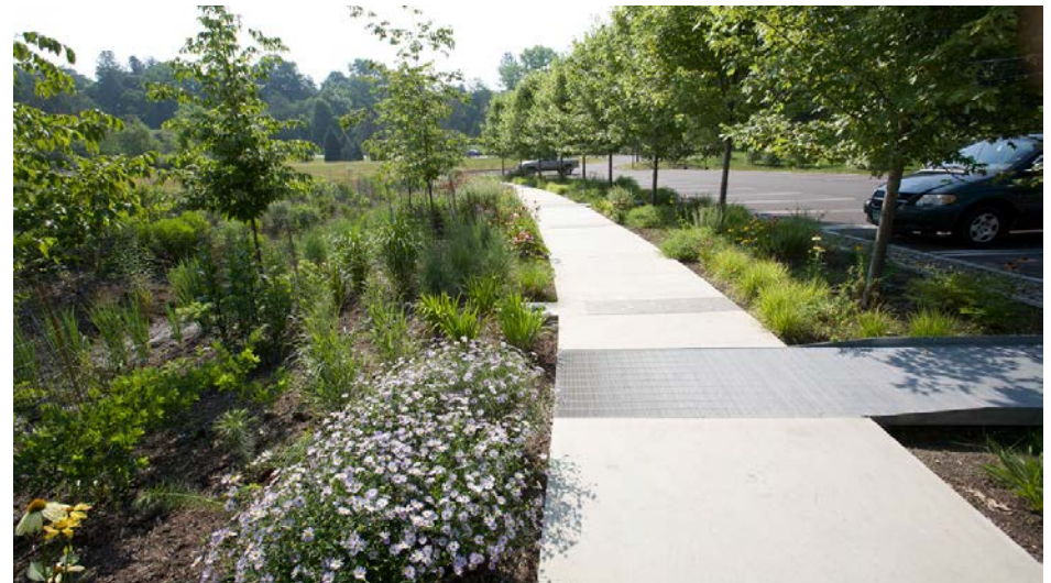
Bioretention swales can be used as green stormwater infrastructure.
