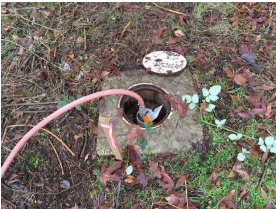
Photo 2 Looking west, red injection hose connected to inflated well plug with fitting installed in well RW-1.
