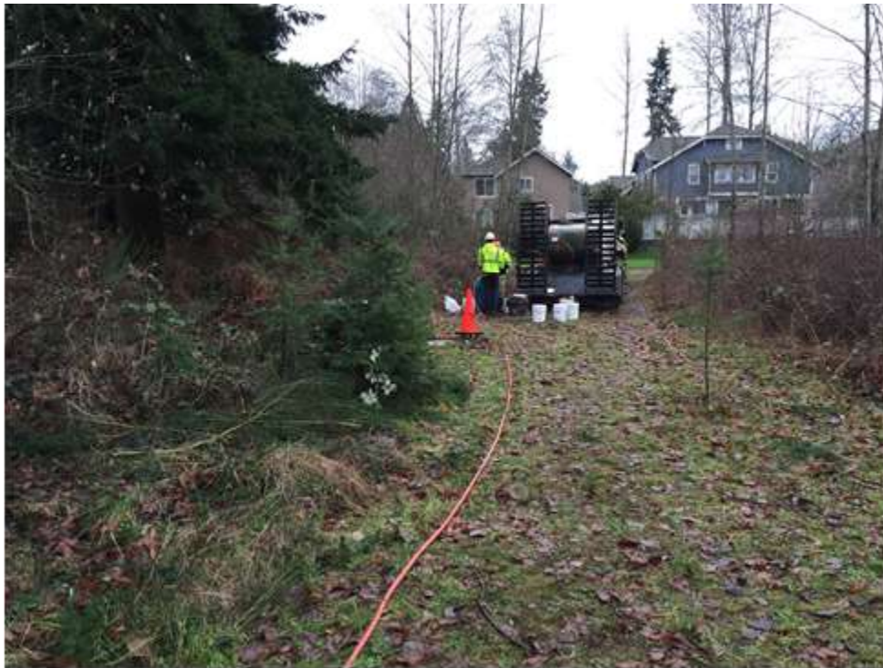
Photo 3 Looking north, Stratus crew at truck and trailer mixing RegenOx for injection into well RW-1.
