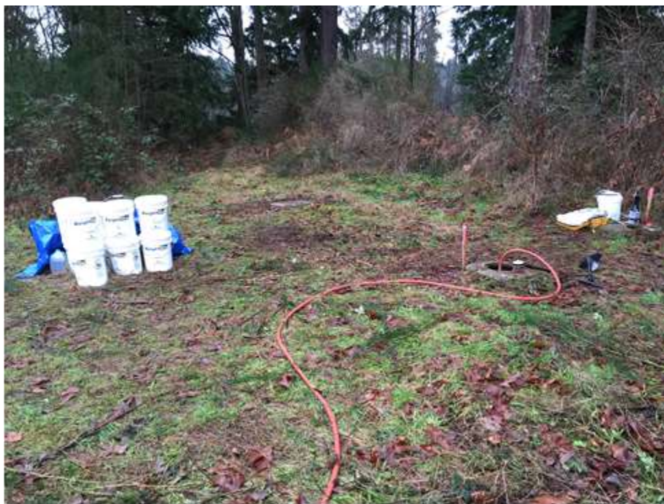
Photo 1 Looking southwest, red injection hose set up at well RW-1, peristaltic pump set up to monitor groundwater at well MW-2A (right background). RegenOx buckets to left.
