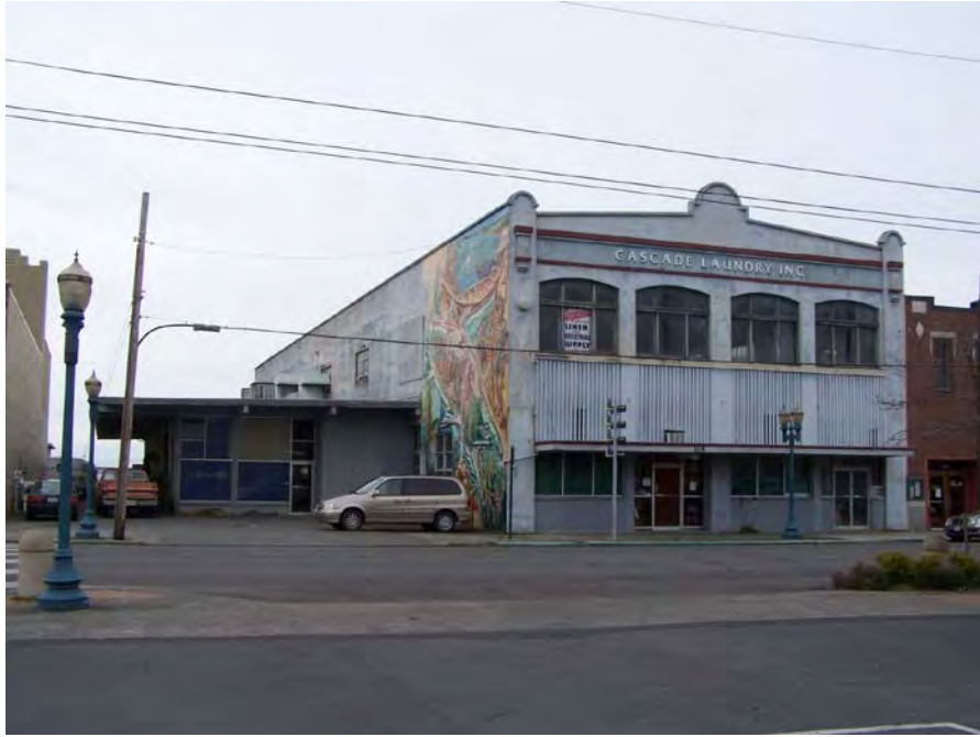
Figure 4. View of the front of the Cascade Laundry building, looking west-northwest across Prospect Street.
