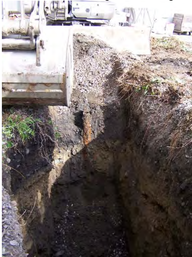
Figure 7. View of test pit #2 in the fill material south of the southwest corner of the building, looking east. The vertical pipe in the far side of the test pit is attached to an underground storage tank.
