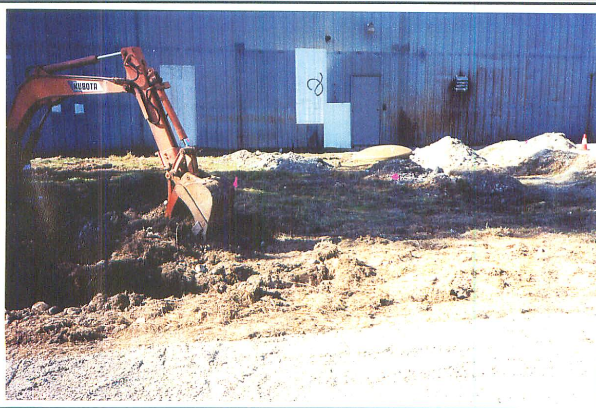
Photo #8: View of the trackhoe excavating the trenches for the purpose of inspecting subsurface soil conditions, facing west towards the Sumner National Auto Parts building. Photo taken on 10/16/02.
