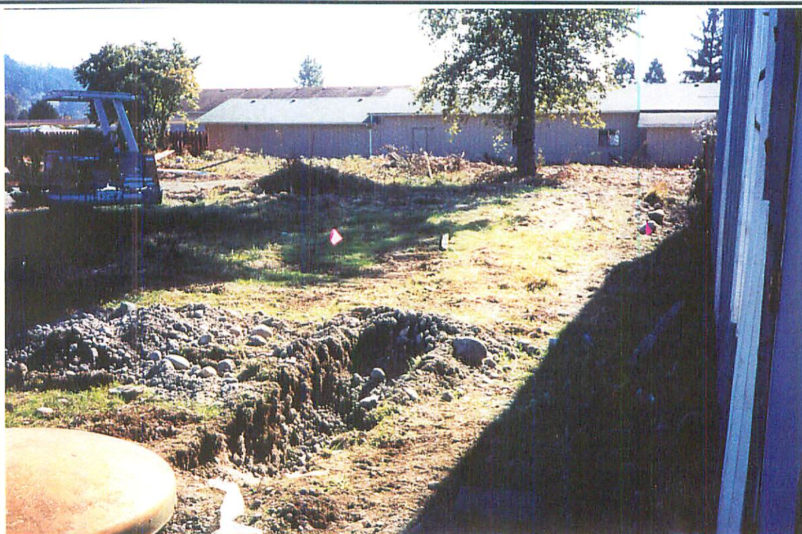
Photo #7: View of the area assessed for reported contaminants, facing south. The ditches were dug for the purpose of collecting subsurface soil samples for analysis. Photo taken on 10/16/02.
