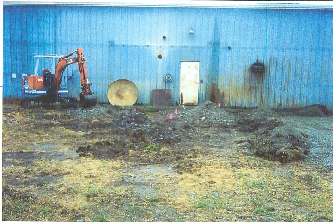
Photo #2: View depicting three (3) excavated trenches and soil sample location flags, facing north toward 60 th Street East. Photo taken on 10/03/02.
