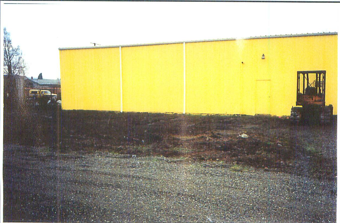
Photo #12: View of the assessed area after the landowner filled and graded in the soil test trenches, facing west. Four to six inches of crushed rock has been placed and graded over some of the assessed area. Photo taken on 12/9/02.
