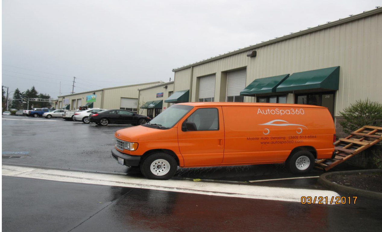
Photo 5: Padden Industrial Park Buildings – from the southeast
