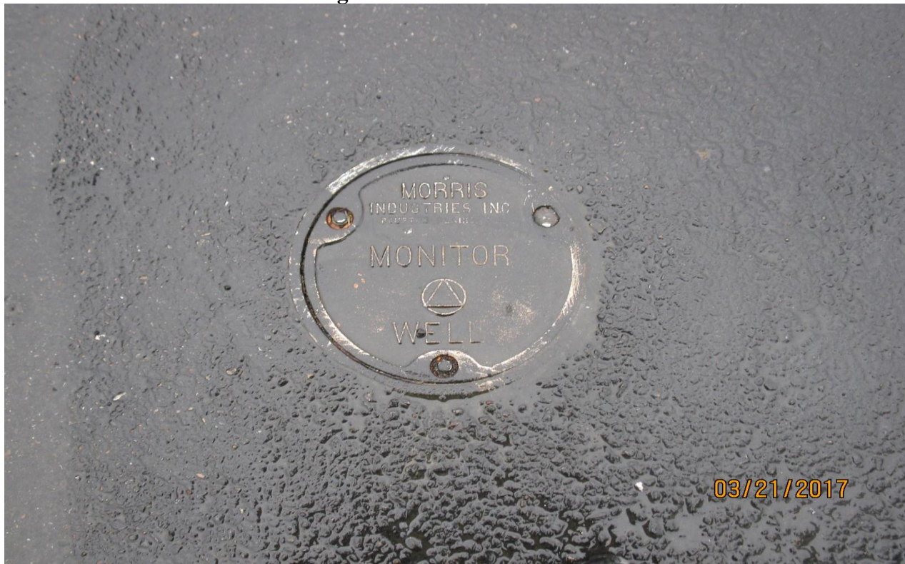
Photo 6: Groundwater Monitoring Well 9b
