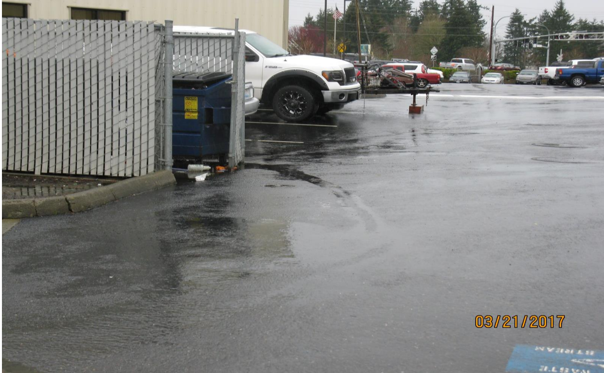
Photo 3: Approximate Area of PCB Soil Contamination Left-in-Place – from the Southwest
