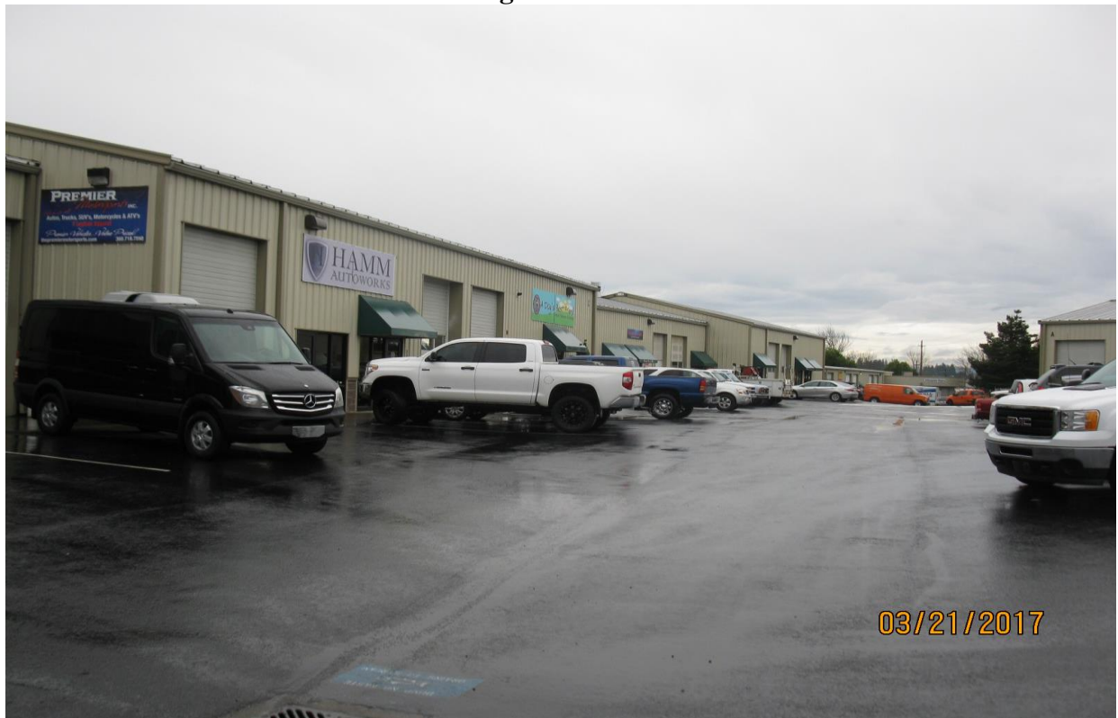
Photo 4: Padden Industrial Park Buildings – from the northwest
