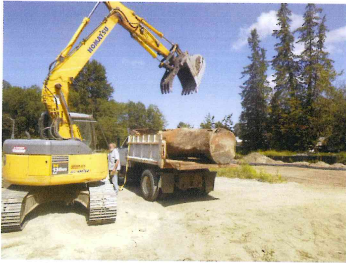
The discovered tank being removed
