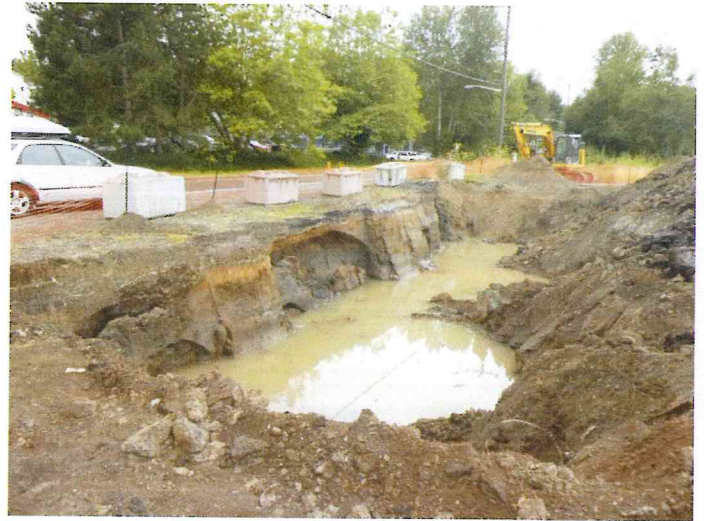
Excavation area from the east looking west on 7/18/2016
