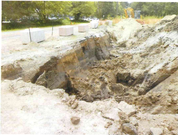
Excavation area from the east looking west on 7/15/2016
