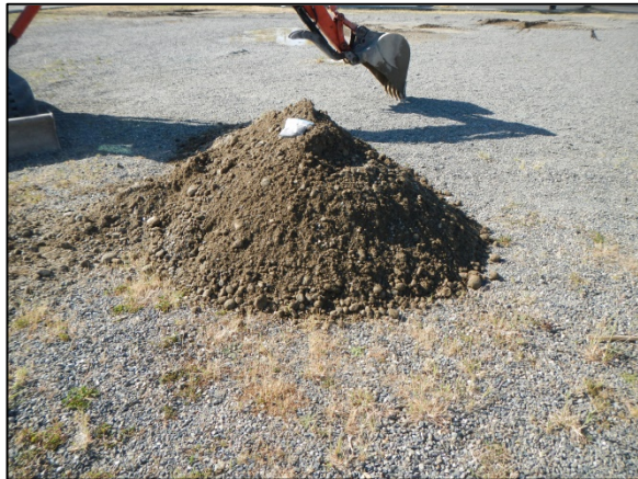
Test Pit TP-4: Spoils pile after completion of test pit.
