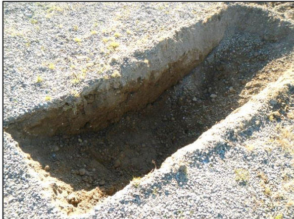
Test Pit TP-2: Test pit during excavation.
