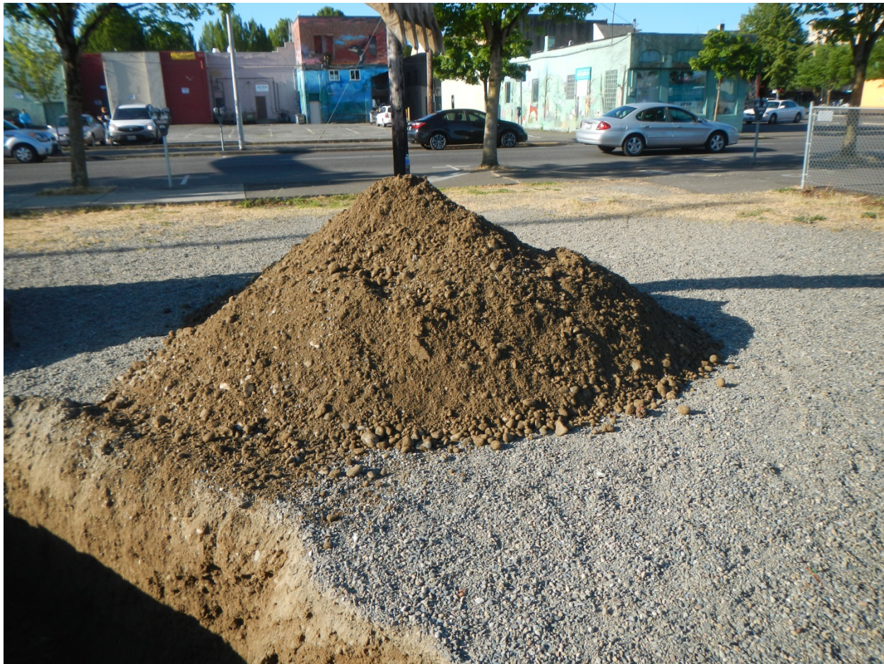
Test Pit TP-1: Spoils pile after completion of test pit excavation.
