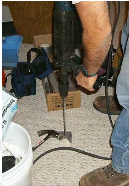
Figure C-1. Drilling through a concrete slab using a rotary hammer drill (EPA 2006)
