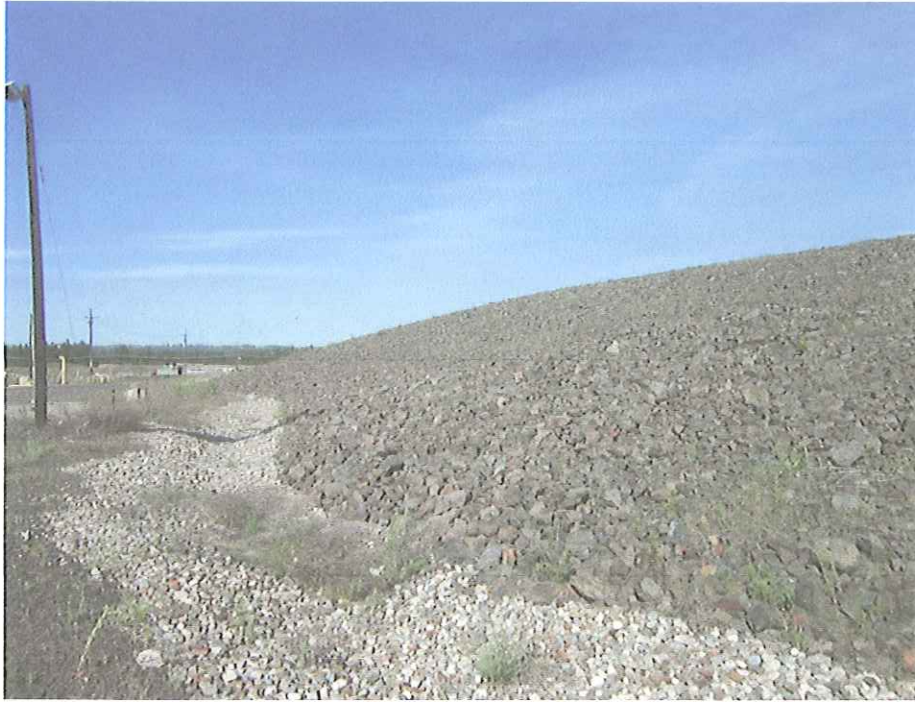
Photo 1: Photograph showing ditch along southeast corner of SPL Pile looking west.
