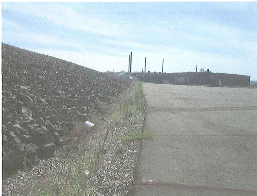
Photo 4: Photograph of SPL west perimeter ditch looking south.
