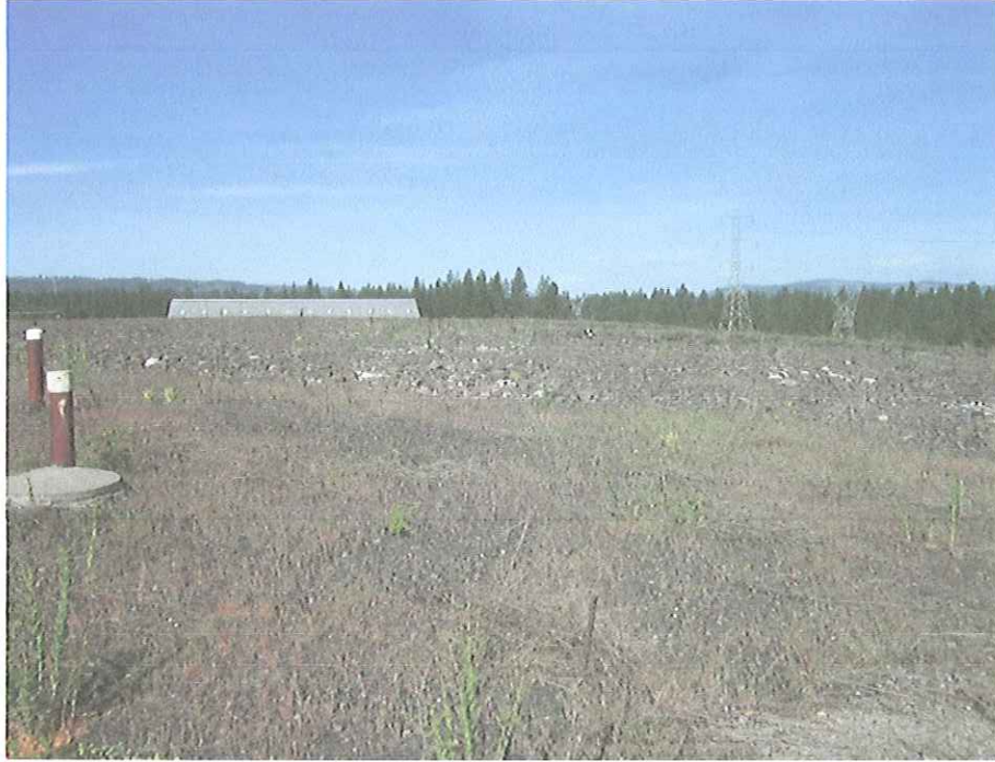
Photo 7: Showing top of of SPL Pile cap looking west.
