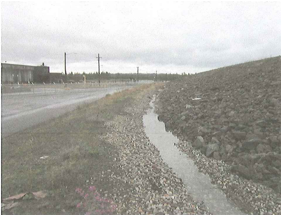
Photo 2: Photograph of perimeter ditch drainage flowing west along south side of SPL pile.
