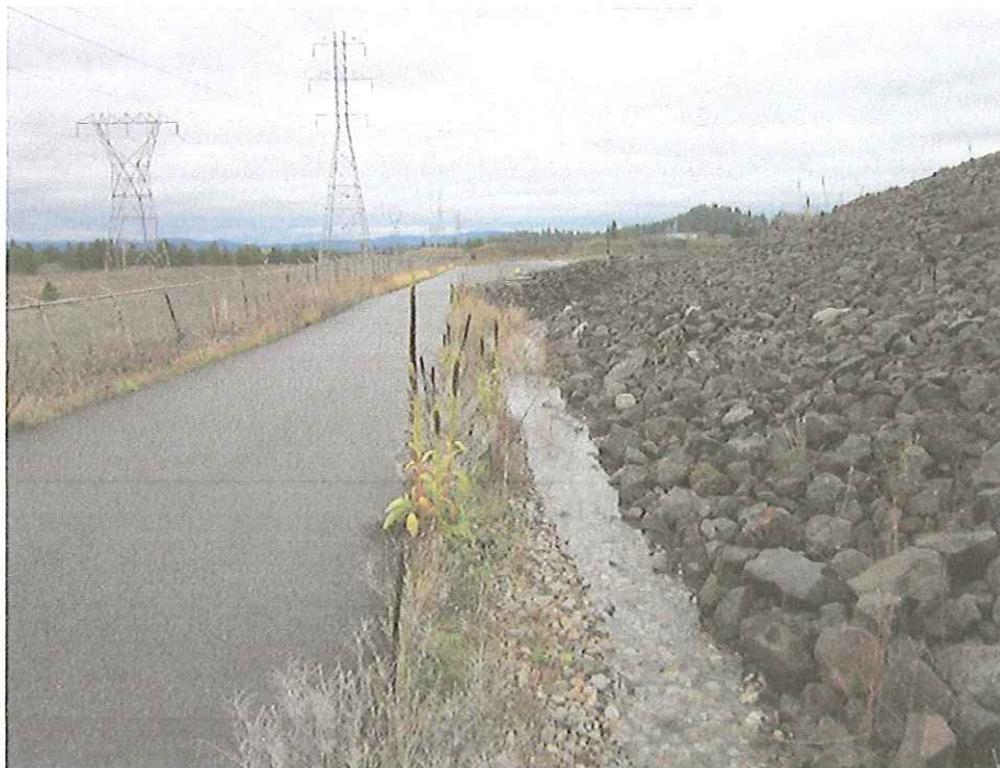
Photo 4: Photograph of end of SPL north perimeter ditch just before entering subsurface drain pipe.
