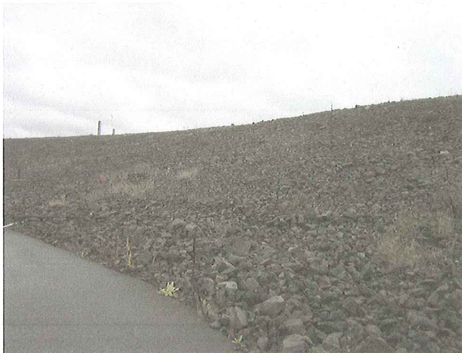
Photo 6: Showing eastern portion of north slope of SPL Pile cap looking southeast.
