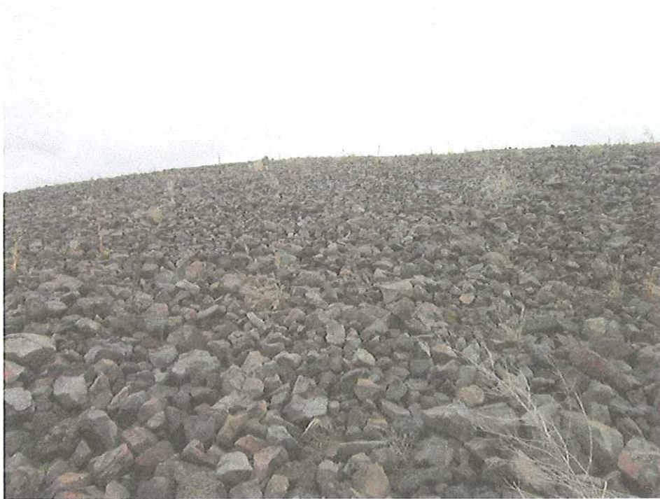
Photo 5: Showing northwest slope of SPL Pile cap.
