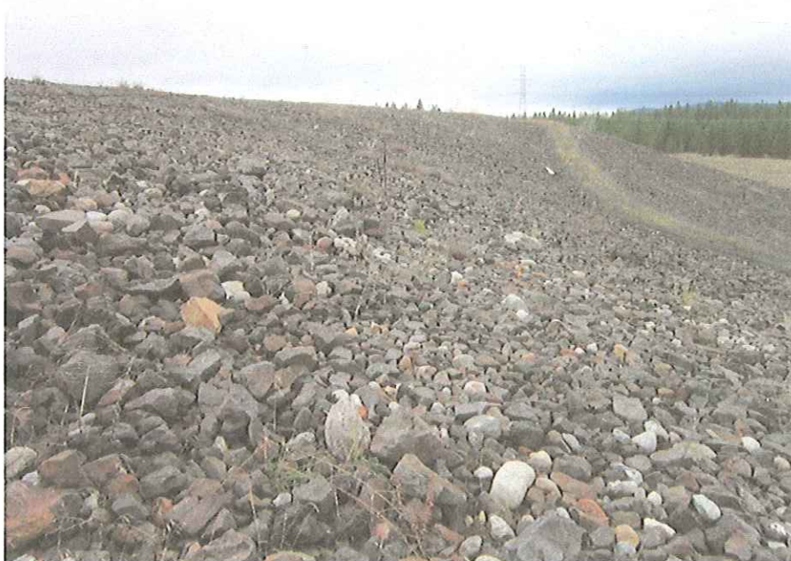
Photo 7: Showing north slope of SPL Pile cap and access road looking west.
