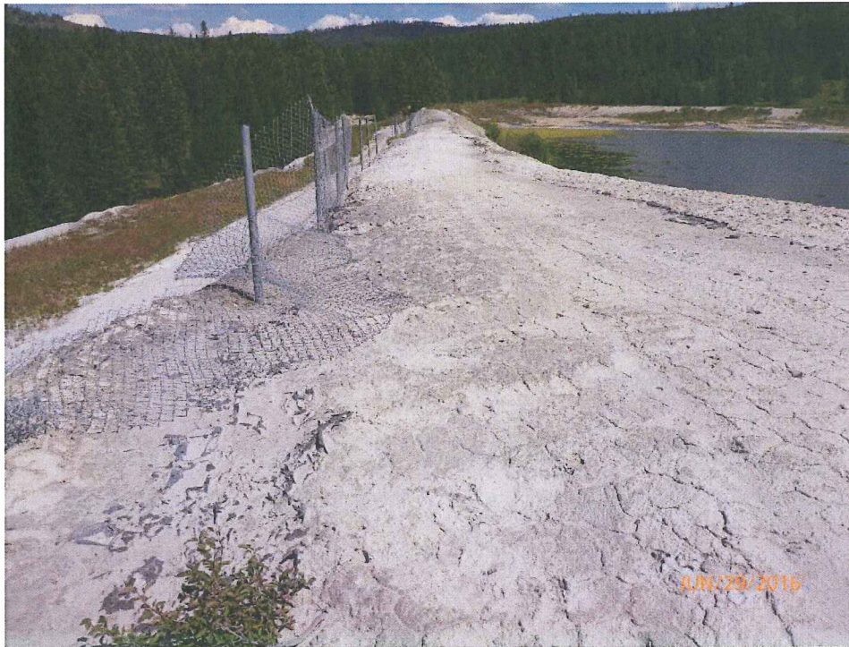
2. East Cell north berm dam crest, looking right (east).
