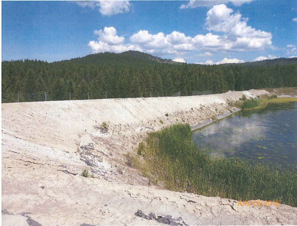
1. East Cell north berm upstream face, looking right (east).
