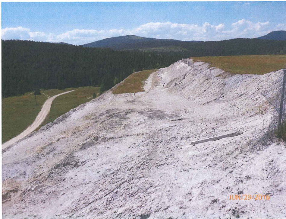
13. West Cell south side downstream face, looking right (west).
