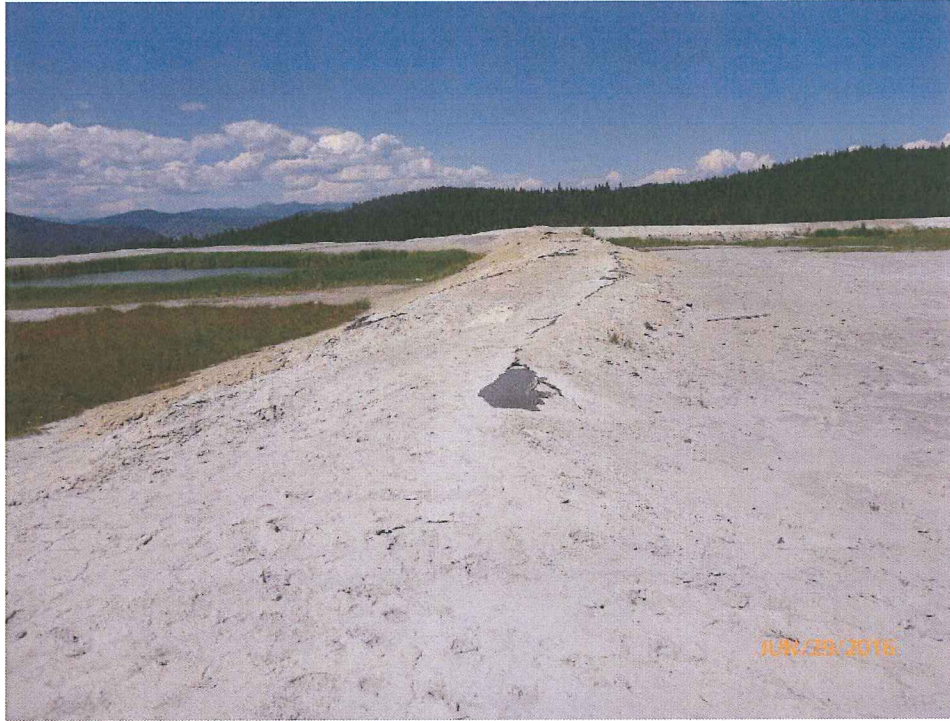
5. Center divider berm, looking north.
