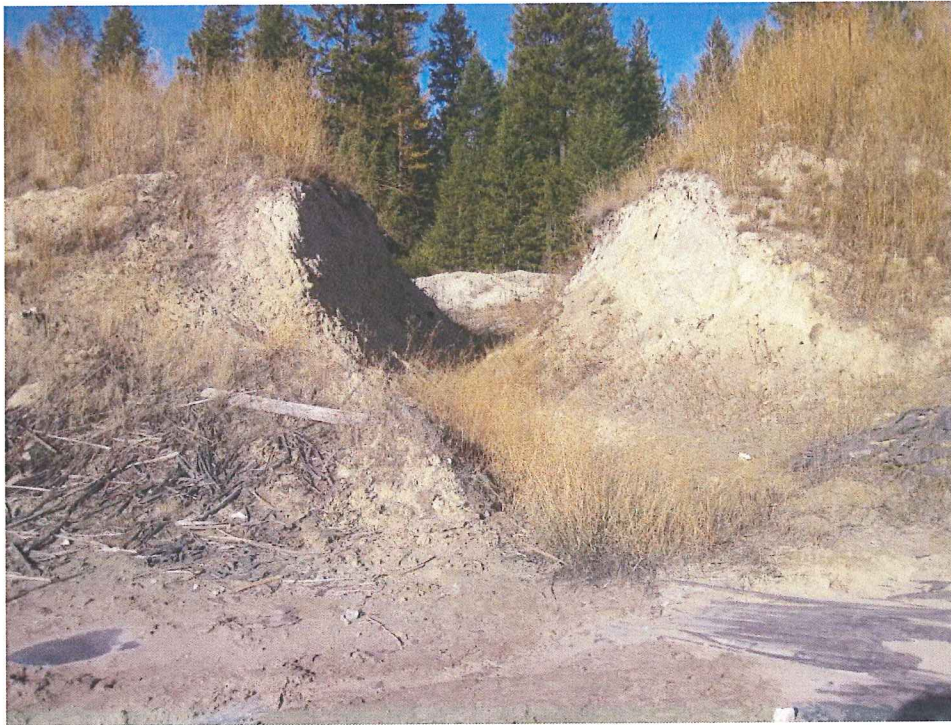
4. East Cell overflow spillway, looking downstream (north) (2011 photo)
