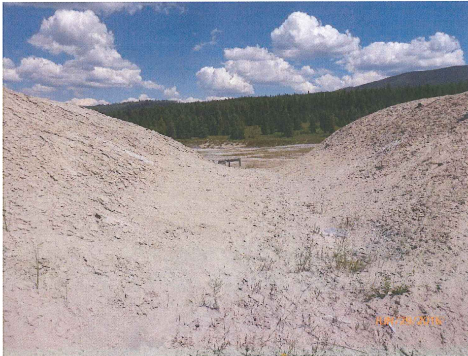
6. Center berm equalizing spillway, looking east.
