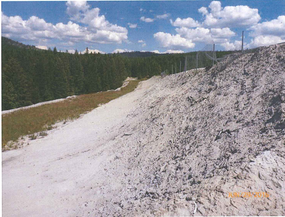
3. East Cell north berm downstream face, looking right (east).
