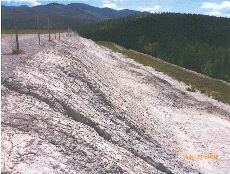
8. West Cell NW side downstream face, looking left.
