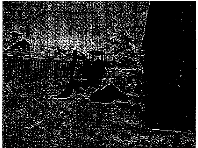
Test pits on souther adjacent property
