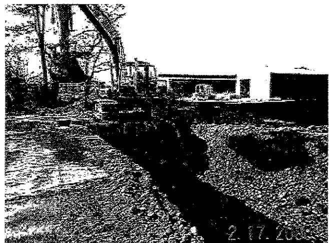
Excavation of Shano ditch
