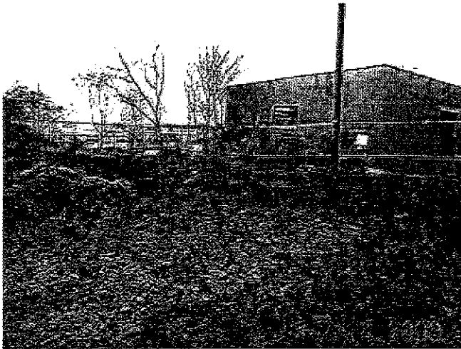
Excavated area grids E6-7, D6-7
