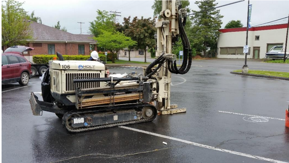
Location of Borehole B2 in the southern parking lot.
