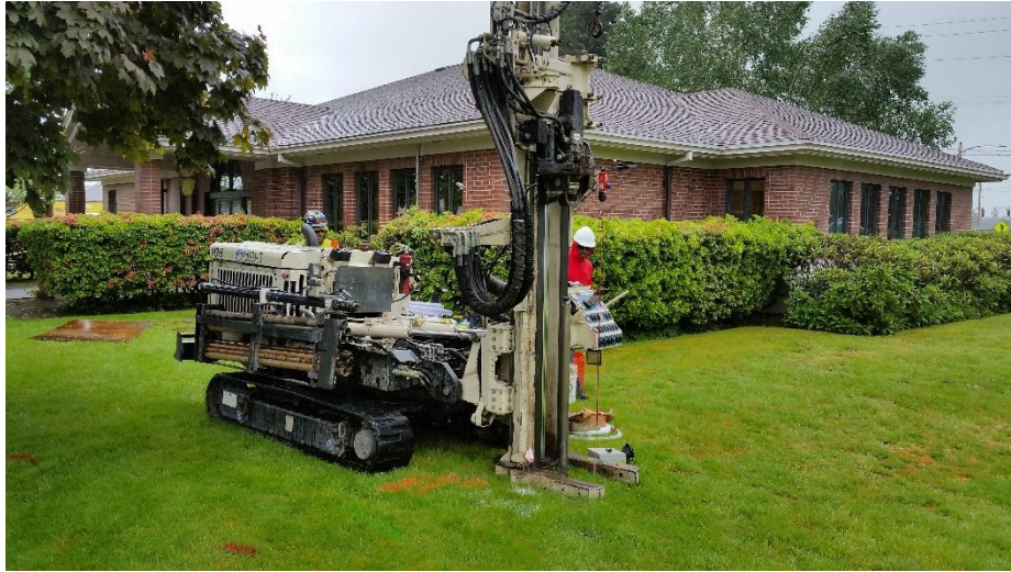
Location of B6 northeast of the building near the former UST's.
