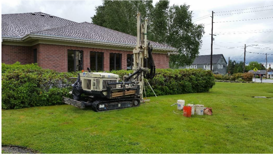
Location of Borehole B8 just north of the building.
