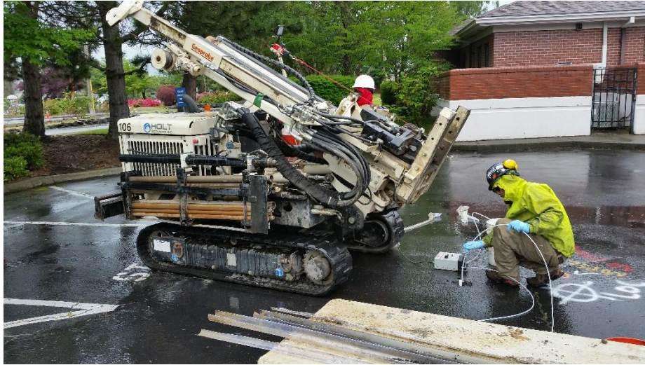
Location of B4 south of the building.
