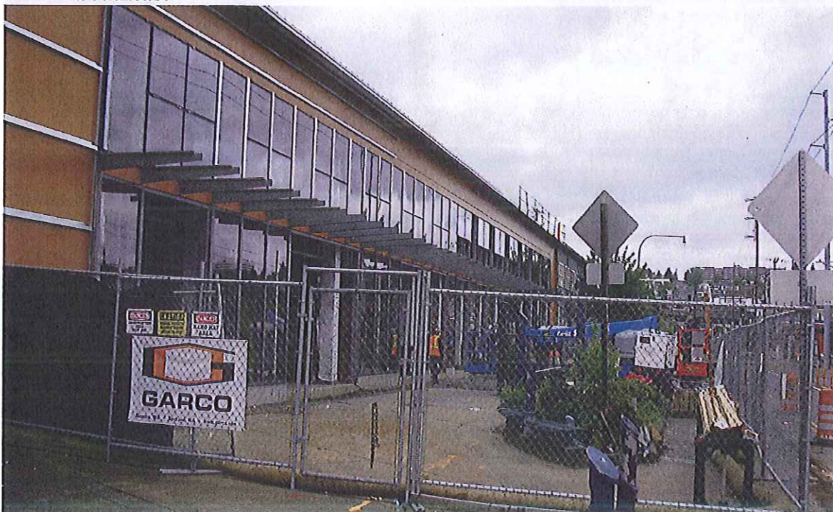
Photo 5: North Side of Building, New Amtrak Train Station Construction—from the Southeast
