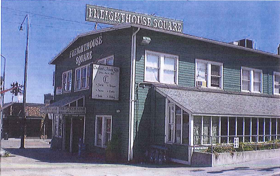
Photo 1: Southwest Corner of Freighthouse Square Building – from the Southwest
