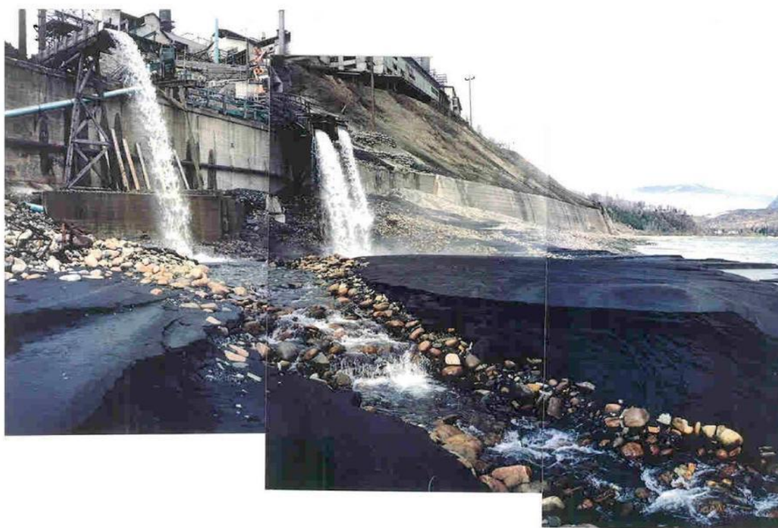
Figure 10: Slag discharge site at Trail in 1992 (from Sigma and Ward, 1992)
