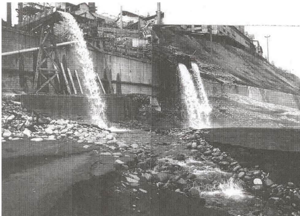
Figure 25. Cominco Metals slag discharge from Sewer #1 on the west bank of the Columbia River just upstream from the Highway 3 bridge (Nener, 1992, p 4, TECK 0715504)
