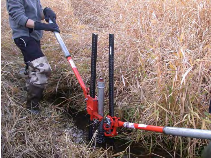
Figure 12 - Decommissioning a steel piezometer with high-lift jacks
