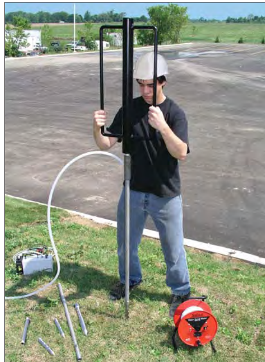
Installing Piezometers with a Manual Slide Hammer
