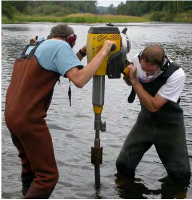
Gas powered jack hammer
