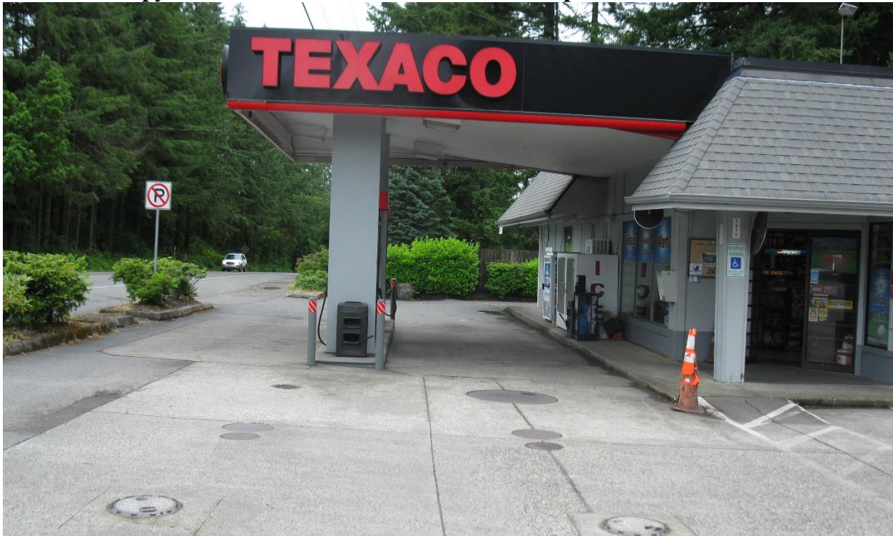
Photo 2: Canopy above the Excavation Area and the Pump Island – From the South
