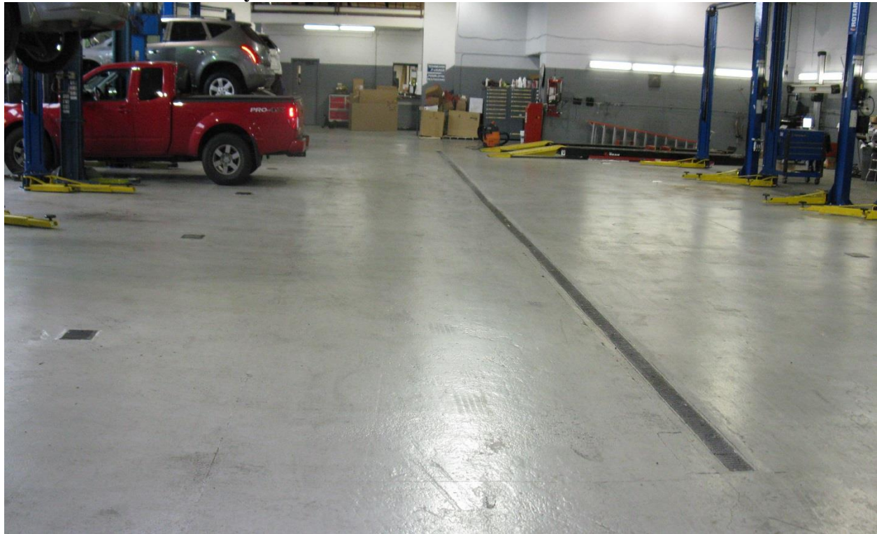
Photo 4: Auto Service Bay – From the South
