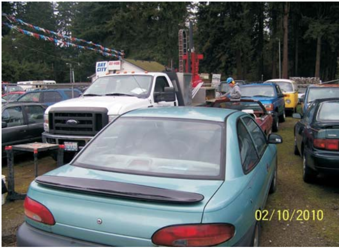
Photo 01 - Setting up on boring B1 west side of former UST Pit
