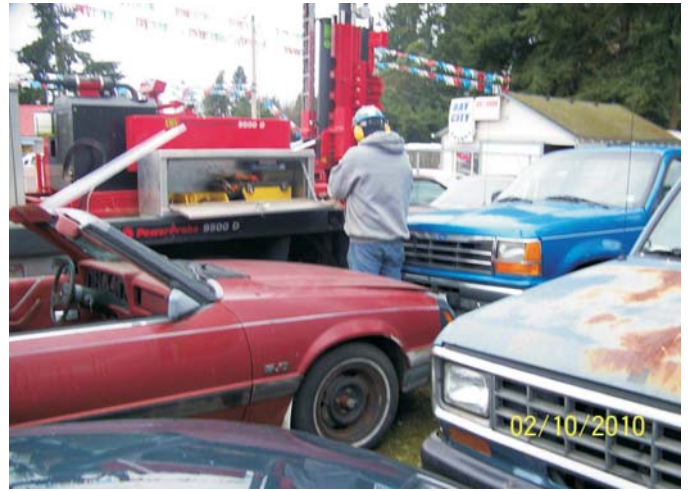
Photo 02 - Drilling on boring B1
