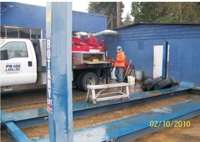
Photo 03 - Drilling on boring B2
