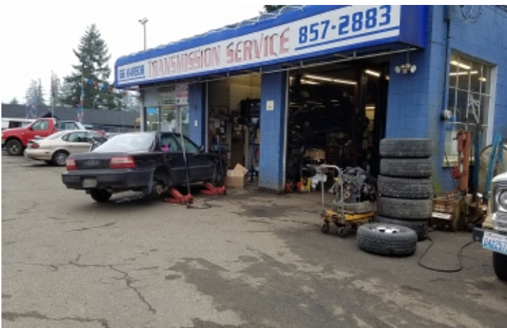
Photograph Five: Exterior Service Bays View SW
