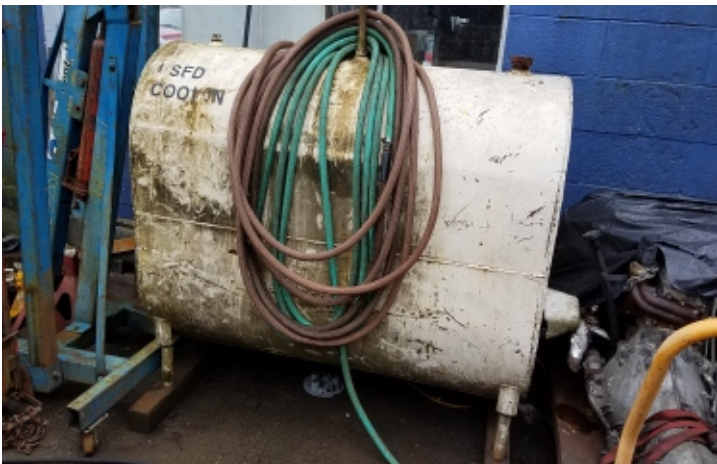
Photograph Eleven: Waste Oil AST.
