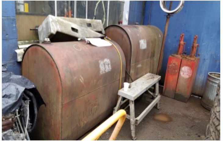
Photograph Ten: Exterior Waste Oil ASTs
