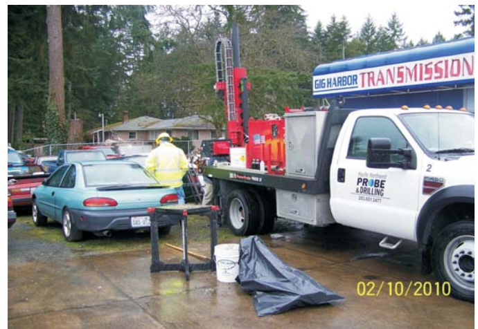
Photo 04 - Drilling on boring B4 north of former UST Pit.
