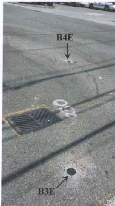
Black circles mark locations of borings B3E and B4E located near the south central portion of the property.
