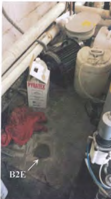
View of the location of boring B2E located near the dry cleaning machine.
