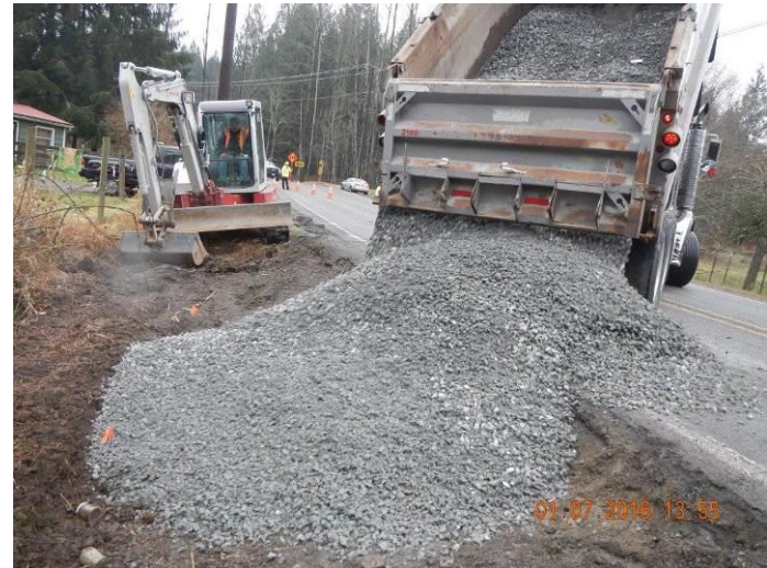
Photo 4: NRC personnel placing backfill material.
