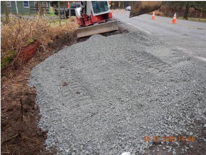
Photo 5: NRC personnel placing backfill material.
