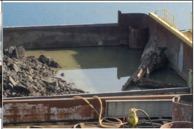
**Comment:** Dewatering haul barge #6 in preparation for sediment offloading. Pumping to tank on barge #BK5.
