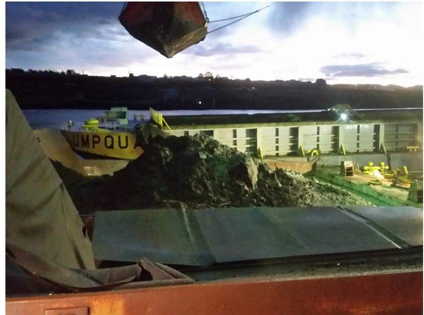
Offloading a haul barge at The Dalles, Oregon. Note the spill apron and fabric to prevent spillage into the river.
