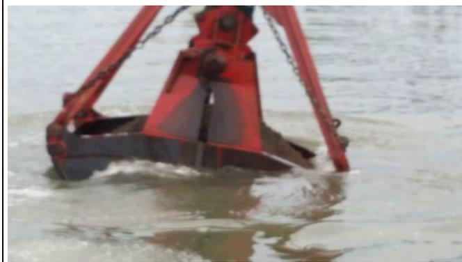
**Comment:** 10 CY Atlas cleanup bucket placing backfill sand.
