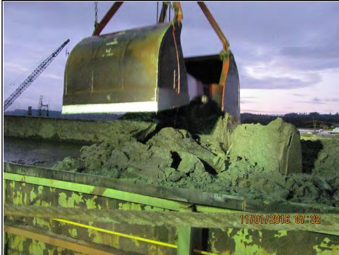
**Comment:** Placing sediments in Scow #6 with rehandling bucket.
