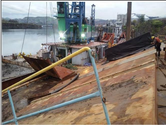
**Comment:** Installing drip plates between dock structure and Barge #BK5
