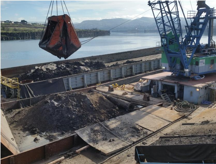
Offloading sediments from a haul barge to the sediment mixing bin. Note the spill plates and splash guards to contain any spillage.
