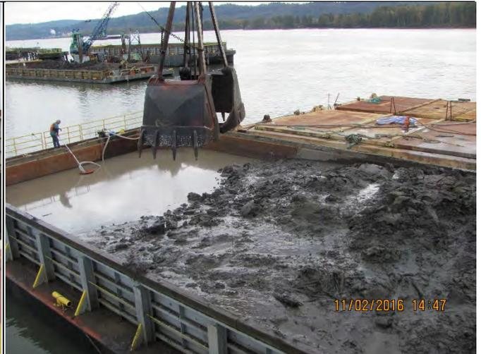
**Comment:** Barge nearly full and pumping free water from the barge into the water management barge.
