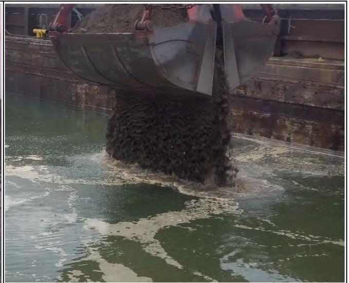
**Comment:** Offloading backfill material from clean fill Barge #31 and placing on shoreward edge of dredge prism.
