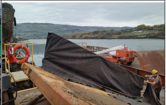
**Comment:** HME installing geotextile fabric as additional splash containment on sides of spill plates
