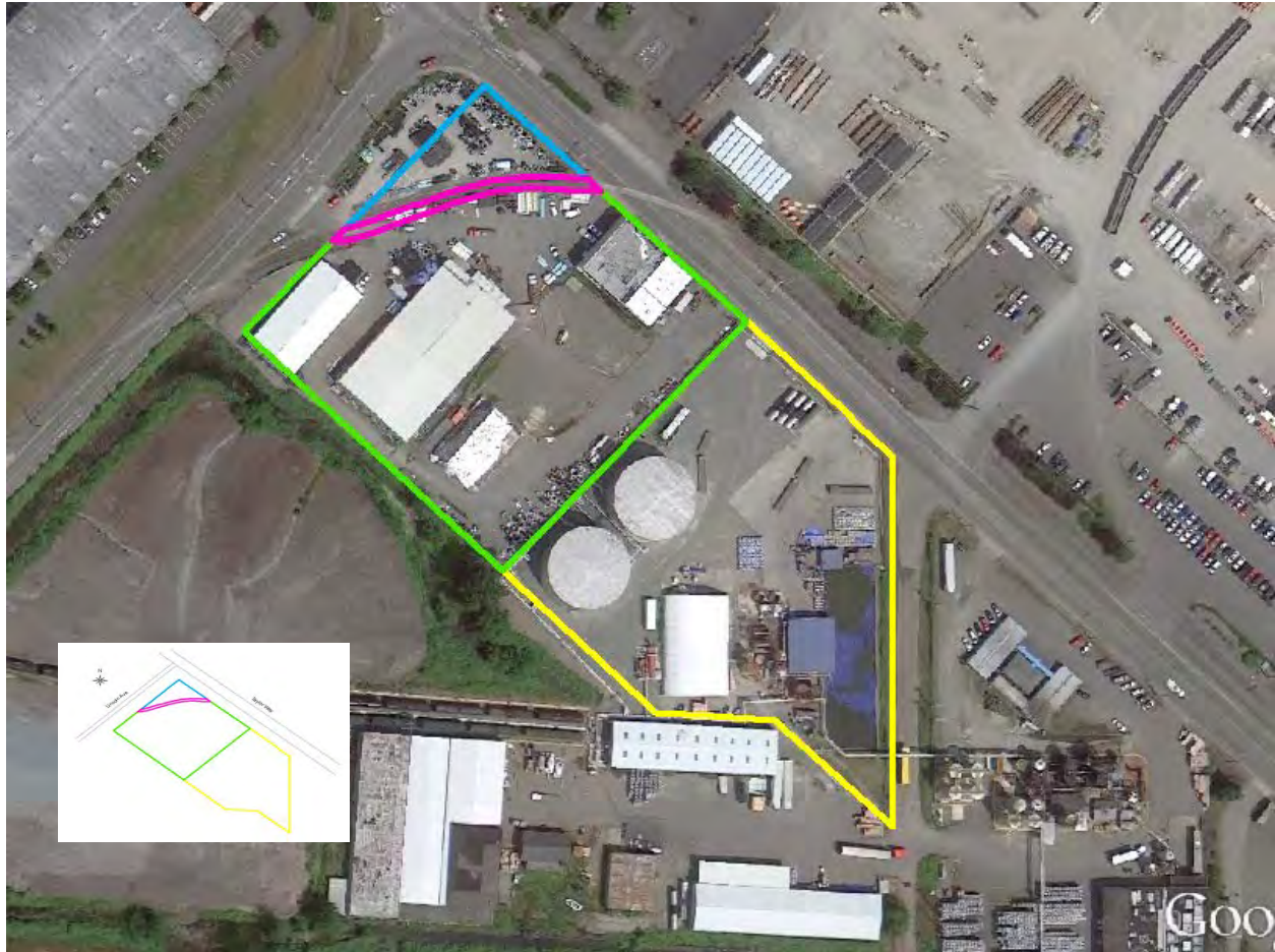
Aerial Photograph 6: The aerial photograph above shows the property as it appeared on July 5, 2012. This photograph shows the results of the on-Property installation of the exposure barrier in the east-southeastern section of the Property, the demolition of Building B and the placement of an exposure barrier in its footprint, and the construction of Building D. The Property remains in the ownership of White Birch Group, LLC., in this configuration. The storage tanks shown on the Gardner-Fields property were constructed in 2011.
