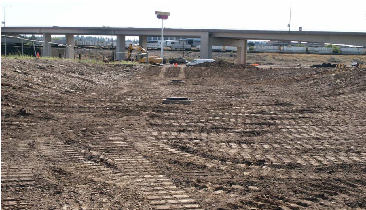
View of north detention basin and new dry wells (looking south).
