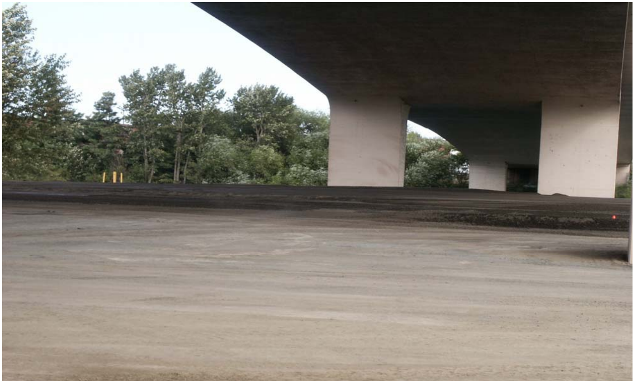
View of top course (looking north-northwest from under bridge).
