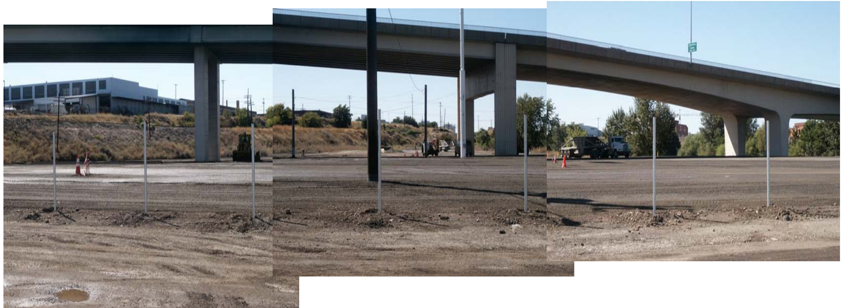
View of re-graded site looking west from Erie Street
