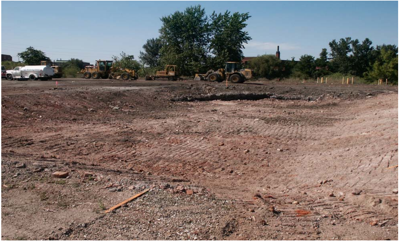
View of west detention basin (looking northwest).
