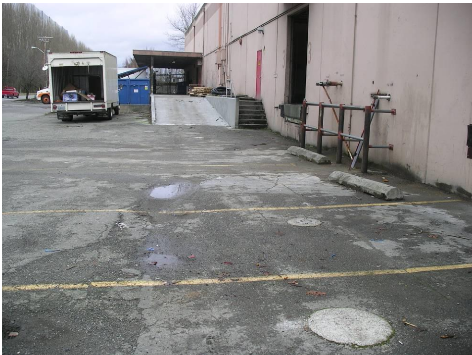
Photo 4: Former Tank Area – from the south
