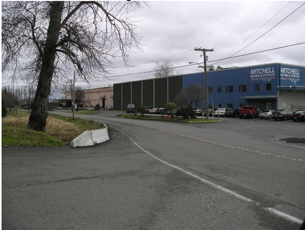
Photo 1: Southwest Side of Building - from the southwest
