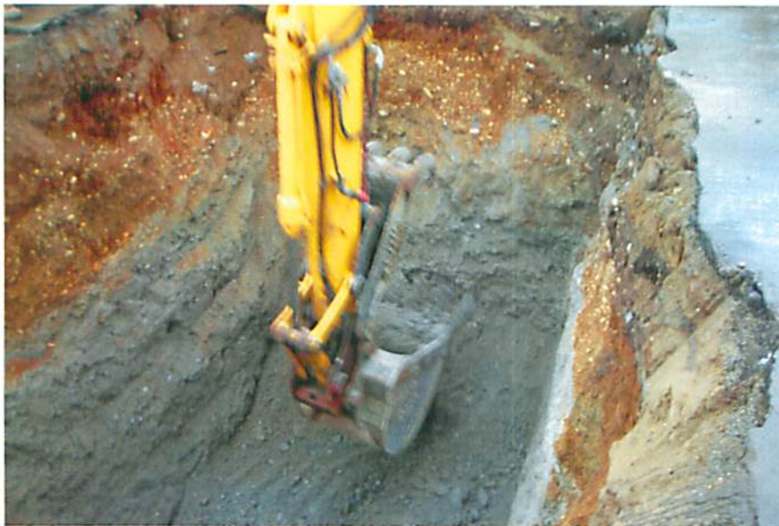
Bottom of tank pit excavation at 20 feet bgs
