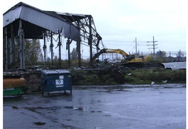
Photograph 54: Demolition of Building 401 (Vanexco building) onto concrete floor slab
