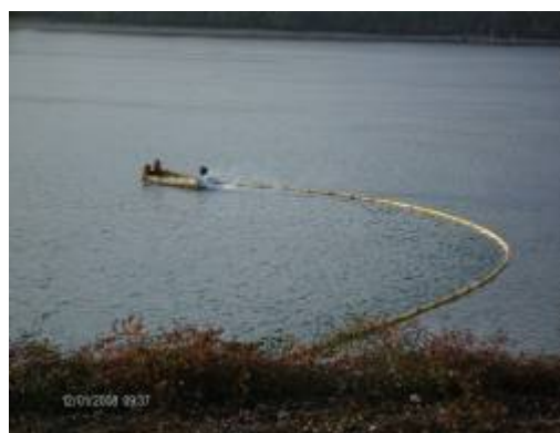
Photograph 4: Debris boom installation
