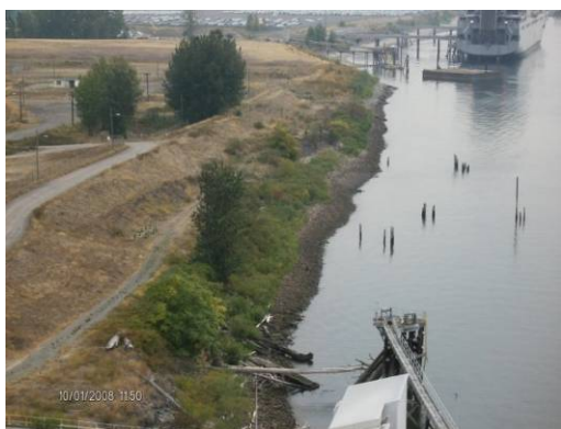
Photograph 33: Dredge areas and piles, taken facing east
