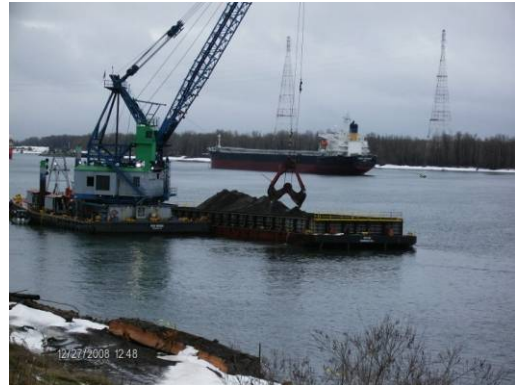
Photograph 36: Dredging, taken facing southeast
