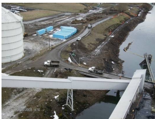
Photograph 22: Transport of dredged material to the North Landfills
