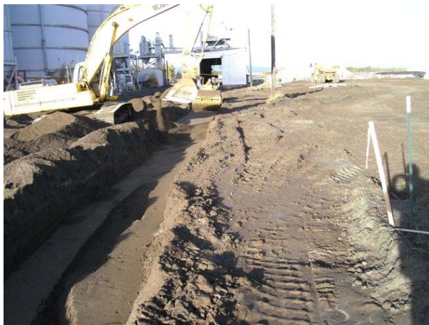
Photograph 60: Storm sewer line removal
