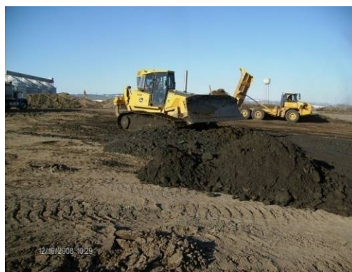
Photograph 23: Spreading of material in the North Landfills
