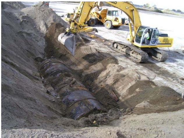
Photograph 47: Soil removal from UST #3
