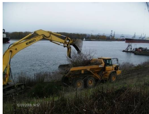
Photograph 8: Clearing and grubbing the shoreline area
