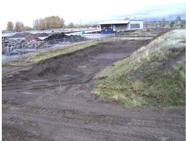
Photograph 49: Removal at SSO 001, 002, and 003
