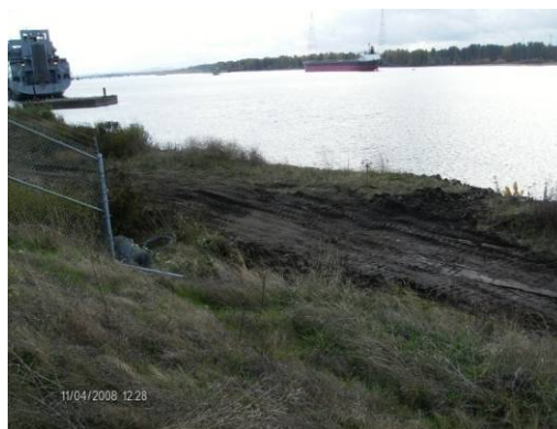
Photograph 6: Removed fencing along the lower levee road
