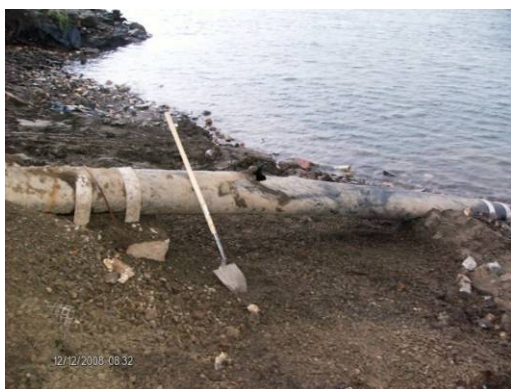
Photograph 12: Damaged outfall
