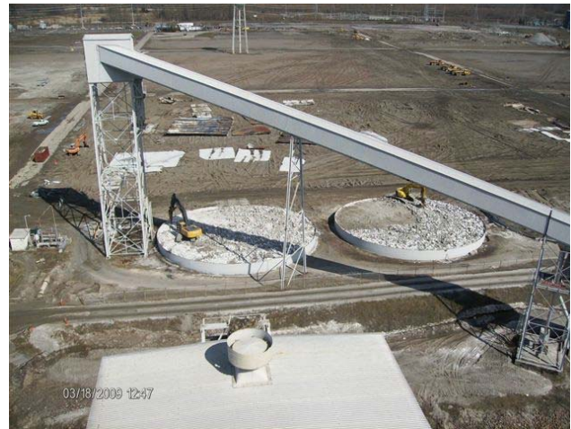
Photograph 56: Demolition of silo foundations
