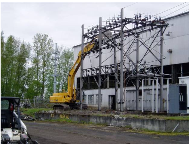
Photograph 53: Demolition of electrical station near Vanexco
