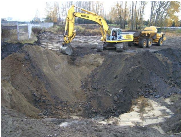
Photograph 64: Excavation of carbon materials
