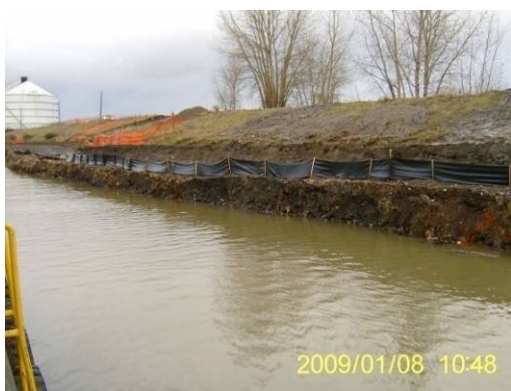
Photograph 3: Erosion fencing
