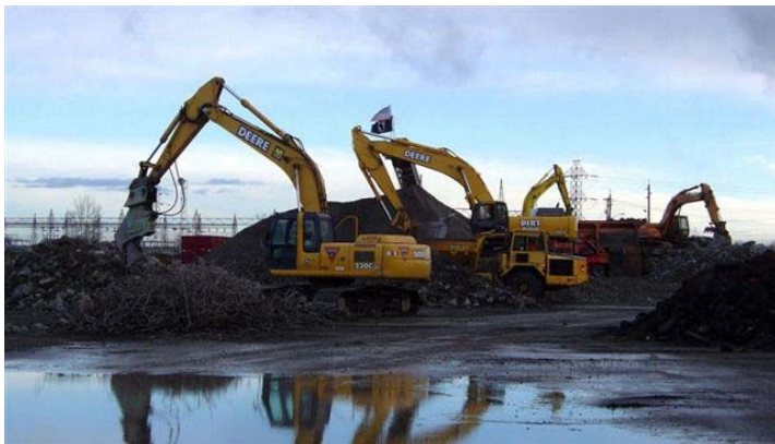
Photograph 57: Crushed concrete piles and relocation activities
