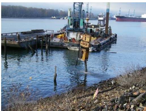
Photograph 16: Pile loosening using vibration Photograph 17: Pile removal
