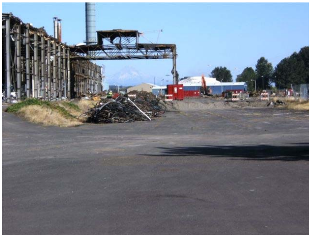
Photograph 51: Demolition of Building 410
