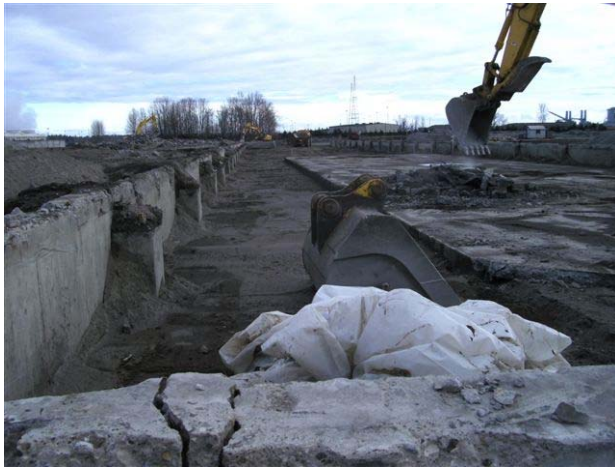
Photograph 58: Excavation under Building 427 to concrete pad
