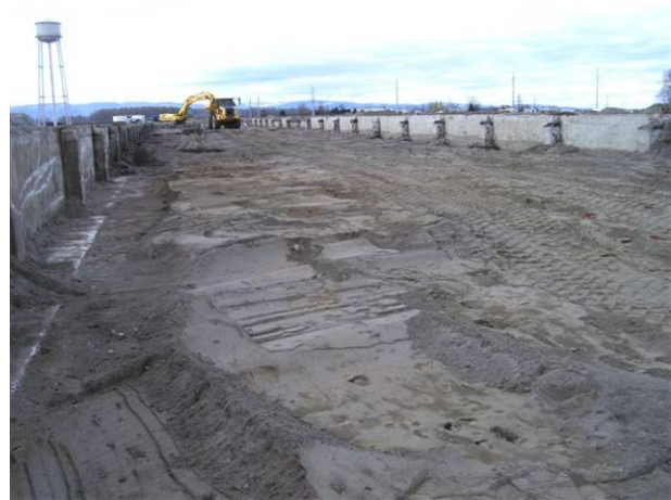
Photograph 59: Excavation under Building 427, looking west
