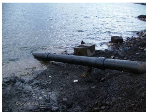
Photograph 13: Repaired outfall
