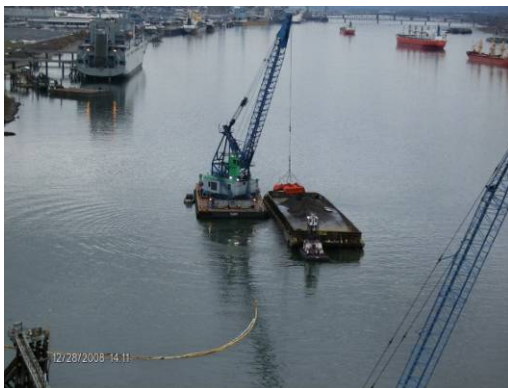
Photograph 37: Dredging with debris boom, taken facing east
