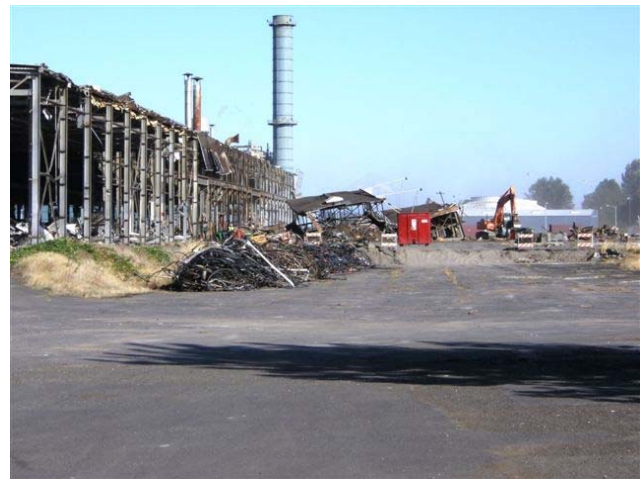
Photograph 52: Demolition of Building 410
