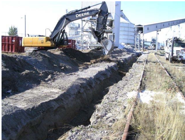
Photograph 62: ASTPT excavation along rail line
