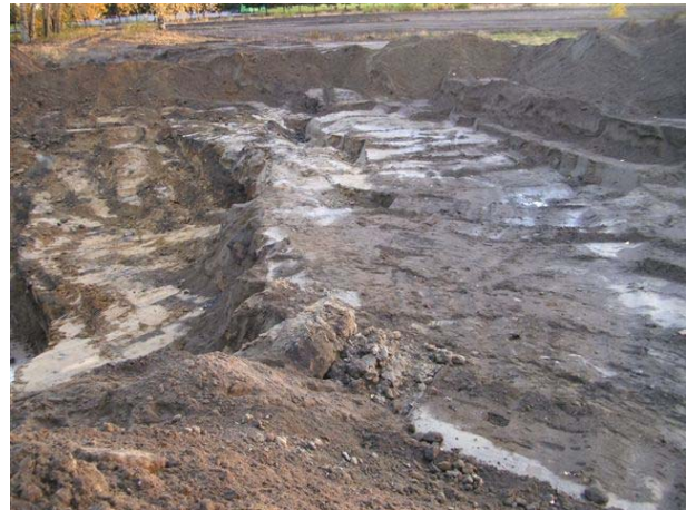
Photograph 65: Completed excavation of the North Soluble Oil area
