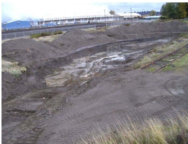
Photograph 50: Removal at SSO 004, 006, and 008
