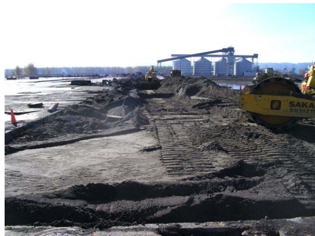
Photograph 61: Storm sewer line excavation backfill and compaction
