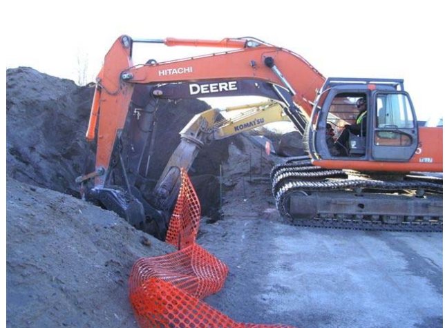
Photograph 48: Removal of UST #3
