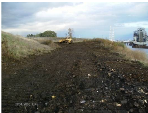
Photograph 5: Grading of the lower levee road
