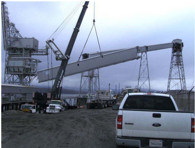
Photograph 55: Crane removing section of ore conveyor
