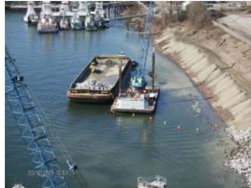
Photograph 2: Installed mesh panel for fish diversion
