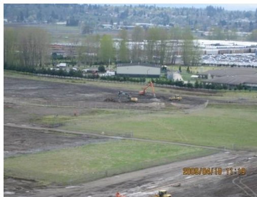
Photograph 25: Final grading of the North and North 2 Landfills
