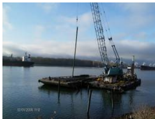
Photograph 16: Pile loosening using vibration Photograph 17: Pile removal
