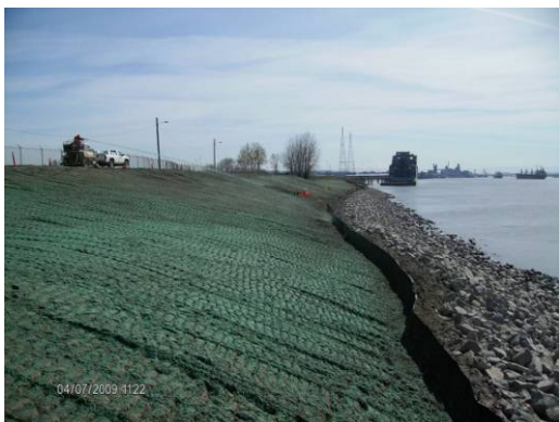
Photograph 24: Hydroseeded shoreline
