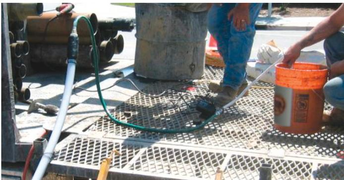
1" diameter Grout Line connected to Grout Adaptor, attached to bottom of CMT.
