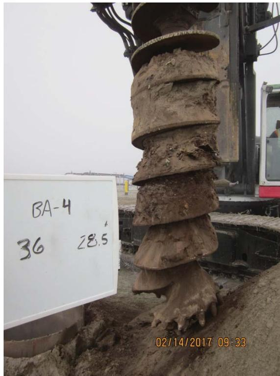
**IMG\_5744:** Recovery 26 to 28.5 ft bgs. Pass No. 1. (2/15)
