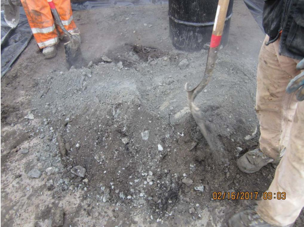
IMG\_5997: Recovery 30.5 to 32 ft bgs. Spread for inspection by Driller's assistant. (3/3)
