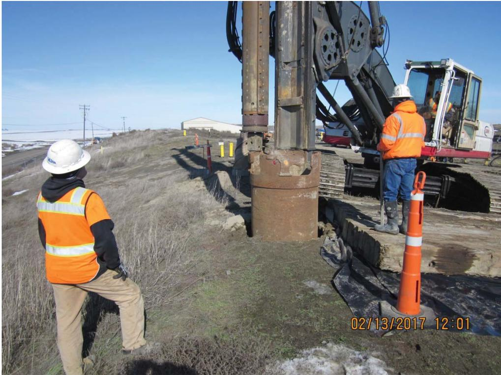
IMG\_5578: Driller setting 48-inch diameter surface casing. (3/3)
