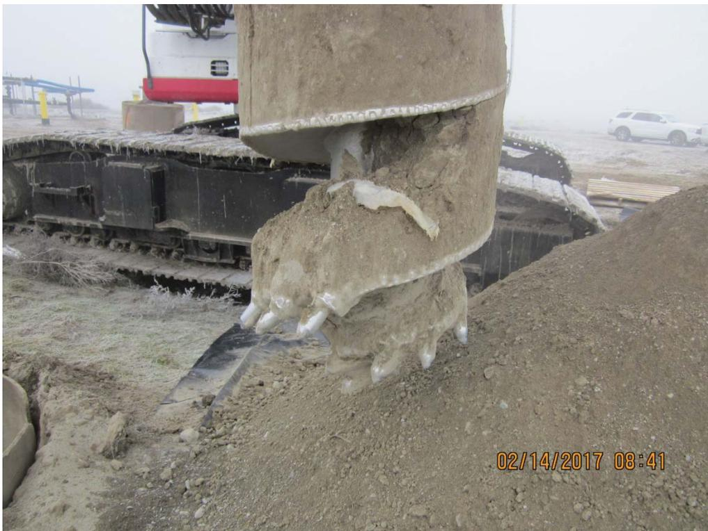
**IMG\_5720:** Recovery 17.5 to 18.5 ft bgs. Piece of Visqueen recovered on bottom flight of auger. (2/2)
