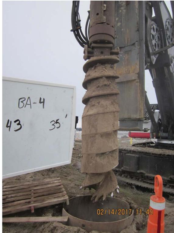
IMG\_5801: Recovery 33.5 to 35 ft bgs. Bottom of boring. (2/4)
