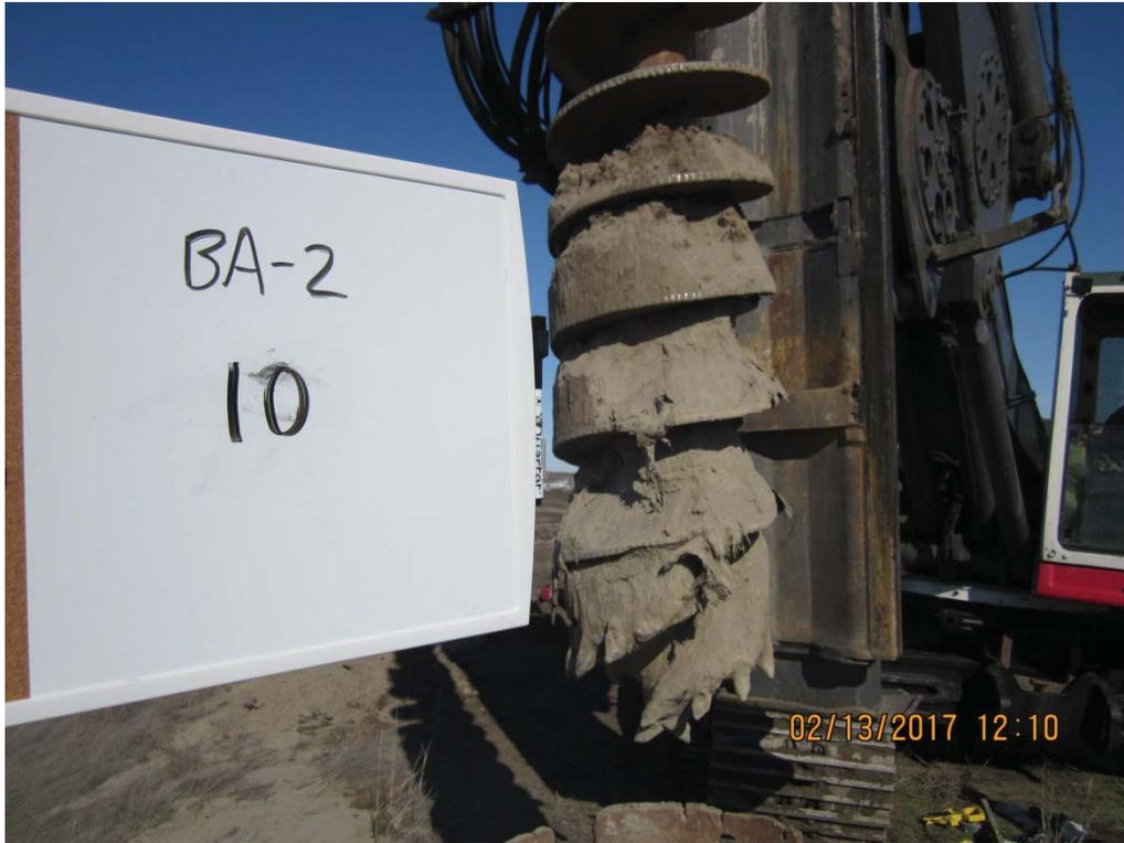
IMG\_5582: Recovery 3 to 5 ft bgs. Piece of Geotextile recovered on auger. Pass No. 5.
