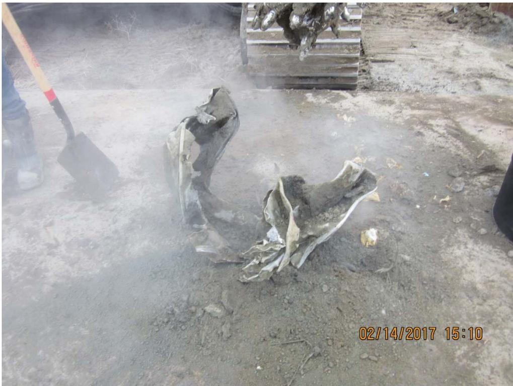
**IMG\_5848:** Recovery 28 to 29 ft bgs. Pass No. 2 Piece of metal drum recovered on auger. (2/2)
