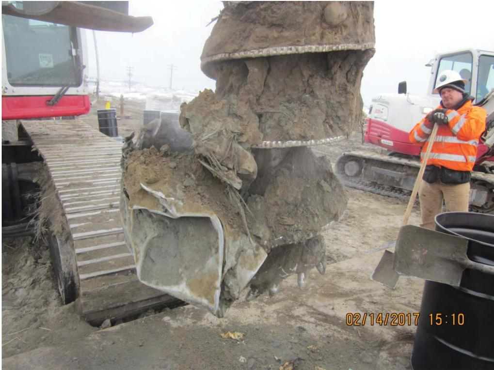
**IMG\_5847:** Recovery 28 to 29 ft bgs. Pass No. 2. Piece of metal drum recovered on auger. (1/2)
