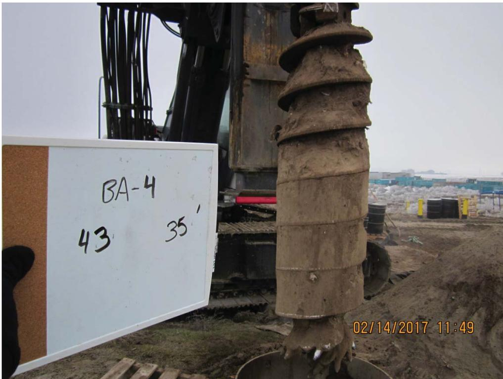
IMG\_5800: Recovery 33.5 to 35 ft bgs. Bottom of boring. (1/4)
