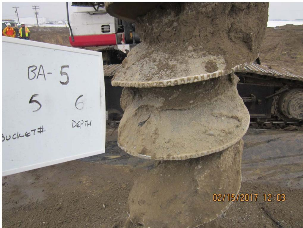
IMG\_5928: Recovery 5 to 6 ft bgs. Pass No. 1. (1/2)
