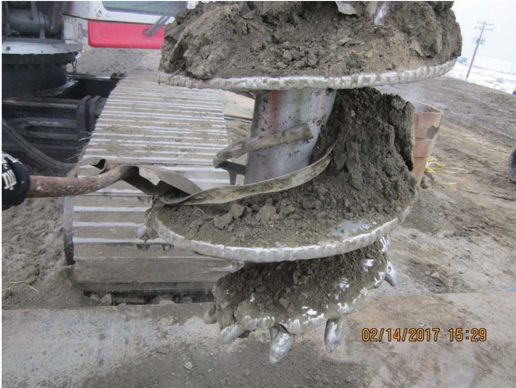
**IMG\_5856:** Recovery 32 to 33 ft bgs. Pass No. 1. Metal fragments recovered. (2/2)
