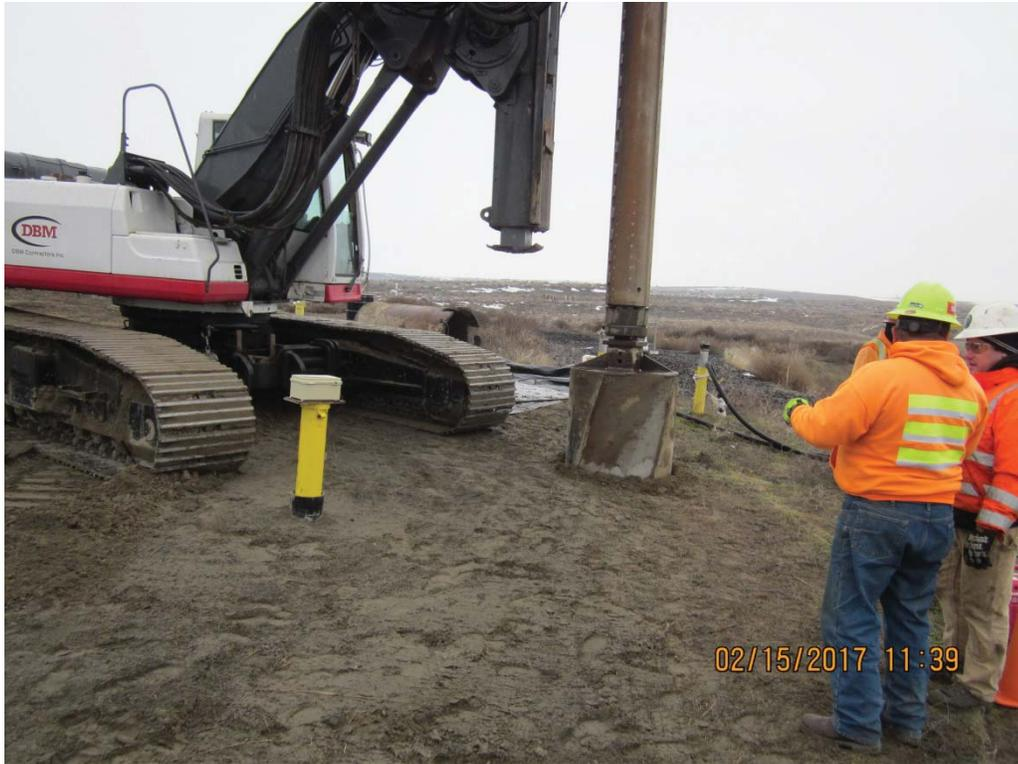
IMG\_5921: Begin drilling and setting fall protection casing at surface. (1/2)
