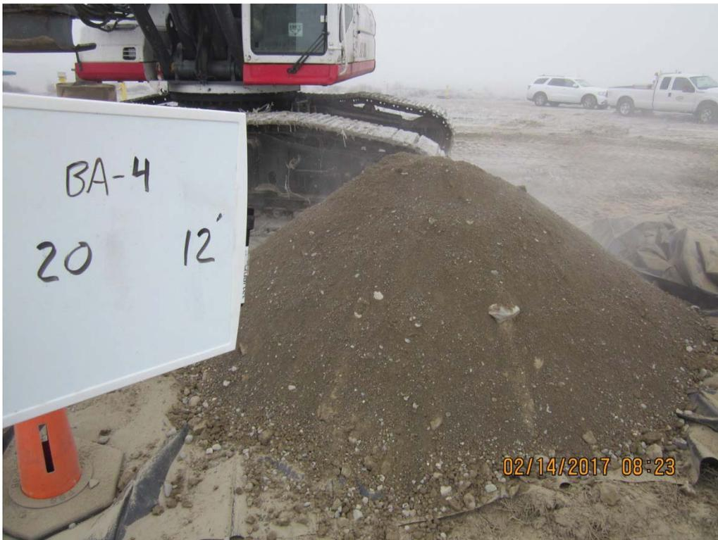
IMG\_5704: Recovery 11 to 12 ft bgs. Pass No. 3. (6/8)
