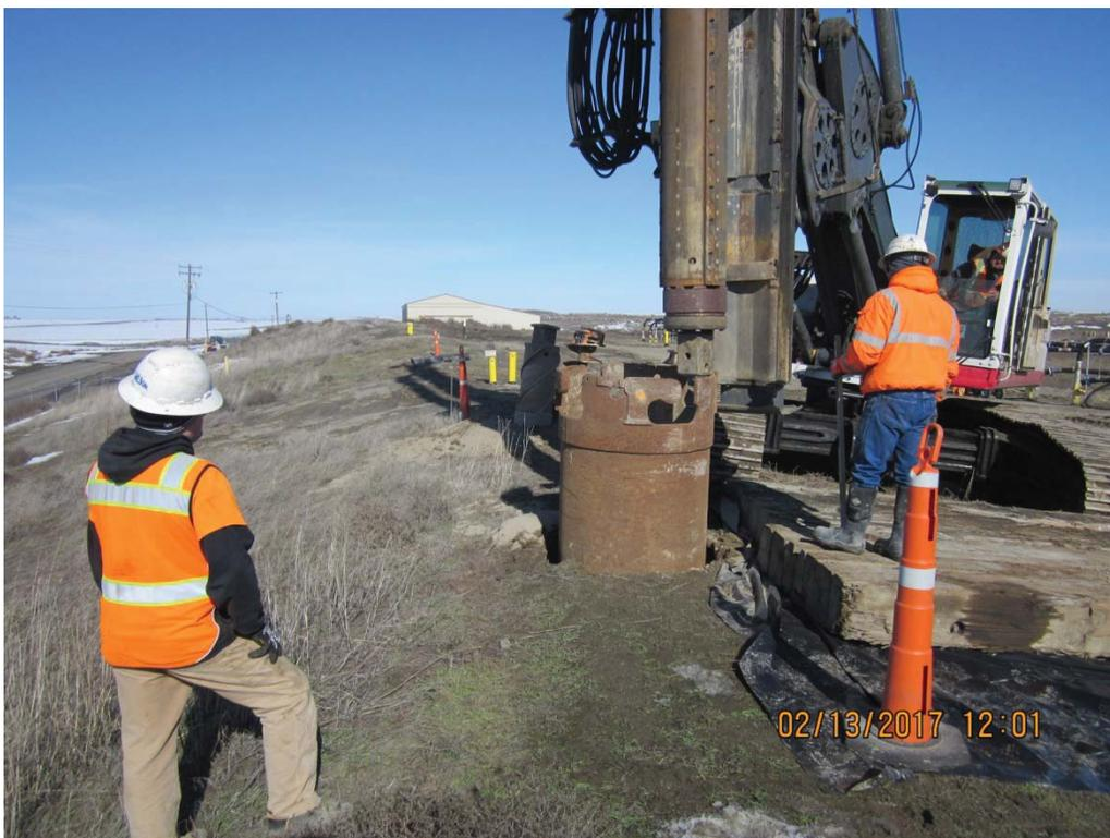
IMG\_5577: Driller setting 48-inch diameter surface casing. (2/3)
