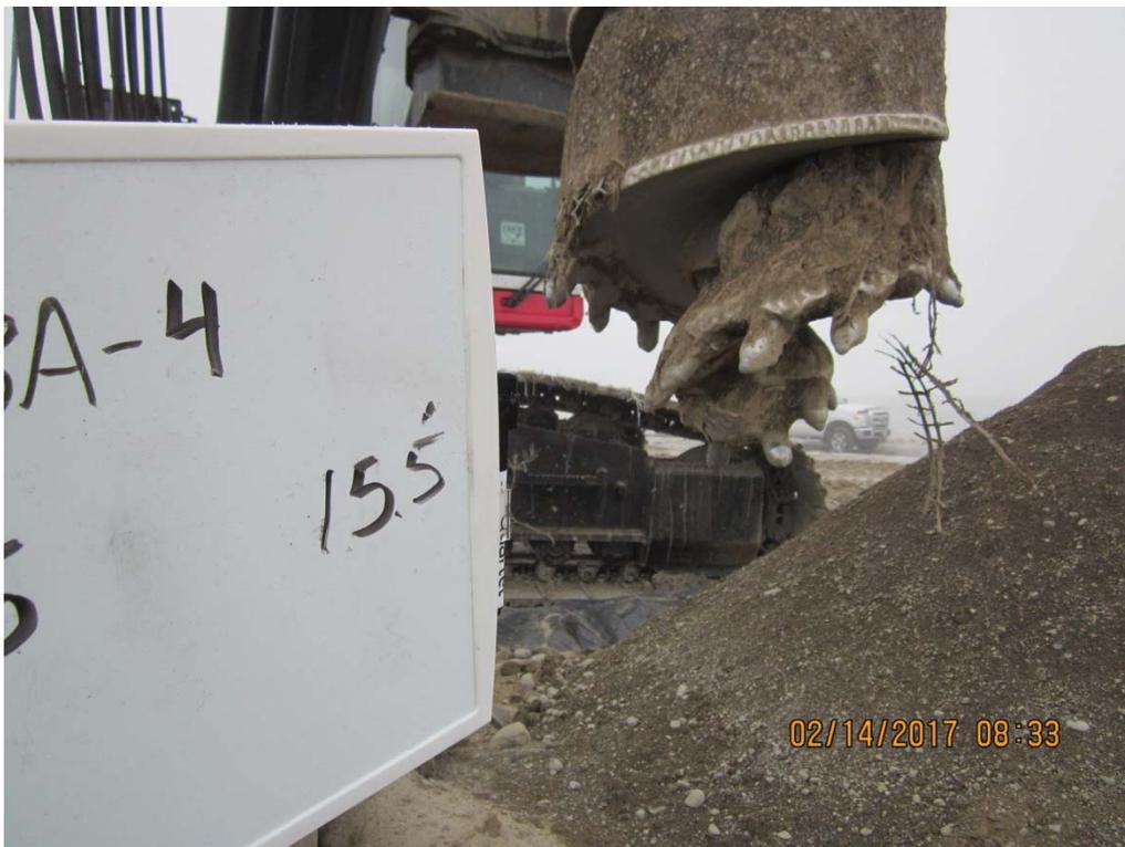
**IMG\_5714:** Recovery 14 to 15.5 ft bgs. Piece of Geogrid recovered on bottom flight of auger. (2/3)
