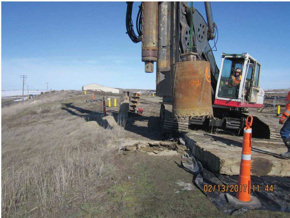
**IMG\_5573:** Driller switching tooling to core barrel prior to setting surface casing.
