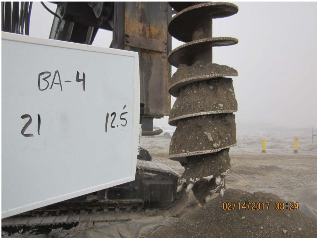
IMG\_5705: Recovery 11 to 12.5 ft bgs. Pass No. 4. (7/8)
