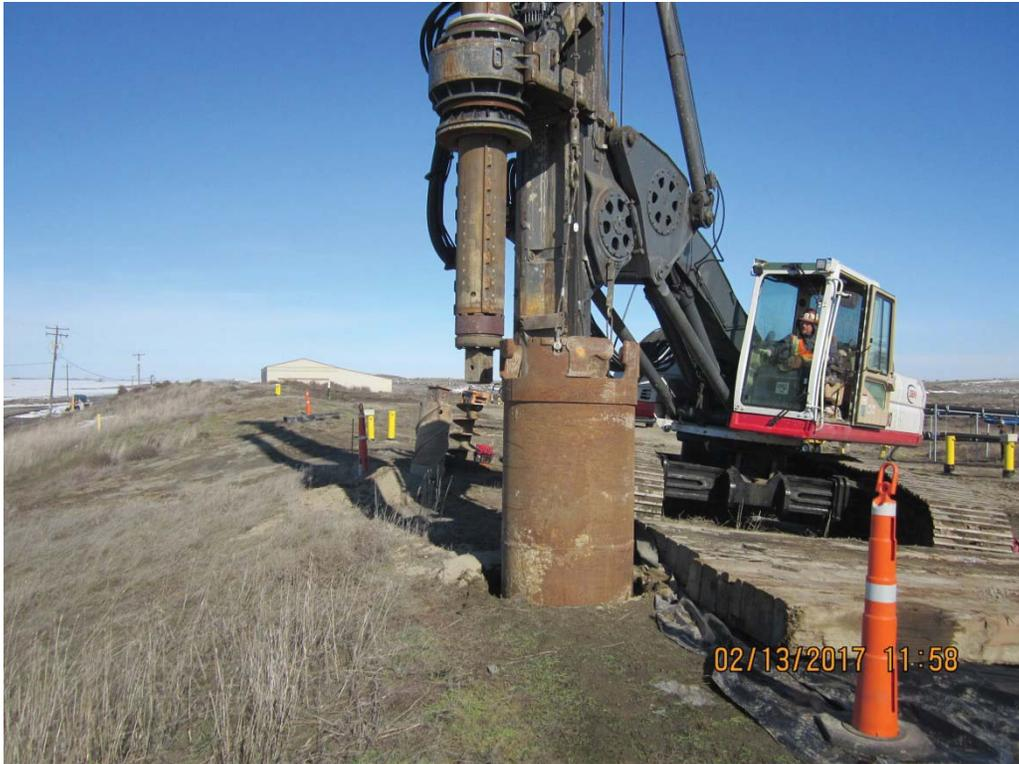
IMG\_5576: Driller setting 48-inch diameter surface casing. (1/3)
