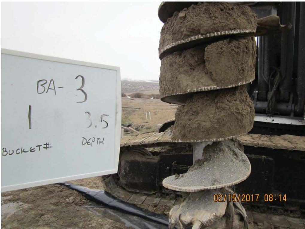
IMG\_5882: Recovery 0 to 3.5 feet (ft) below ground surface (bgs.). Piece of Geotextile recovered on bottom flight of auger.
