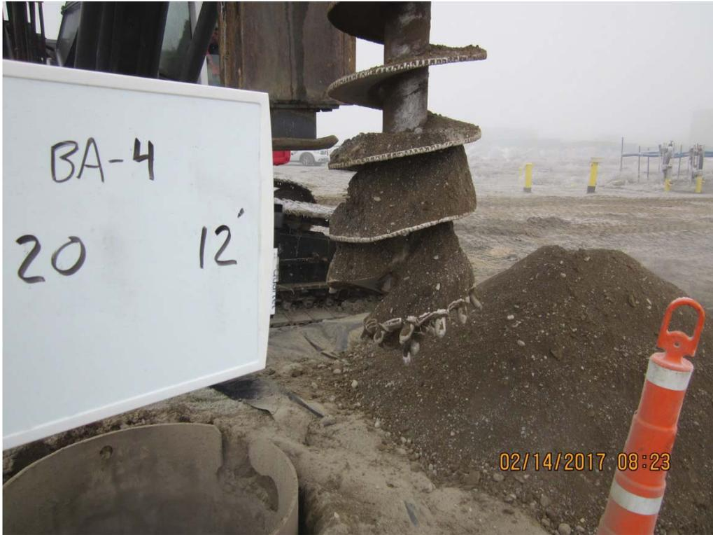
IMG\_5703: Recovery 11 to 12 ft bgs. Pass No. 3. (5/8)
