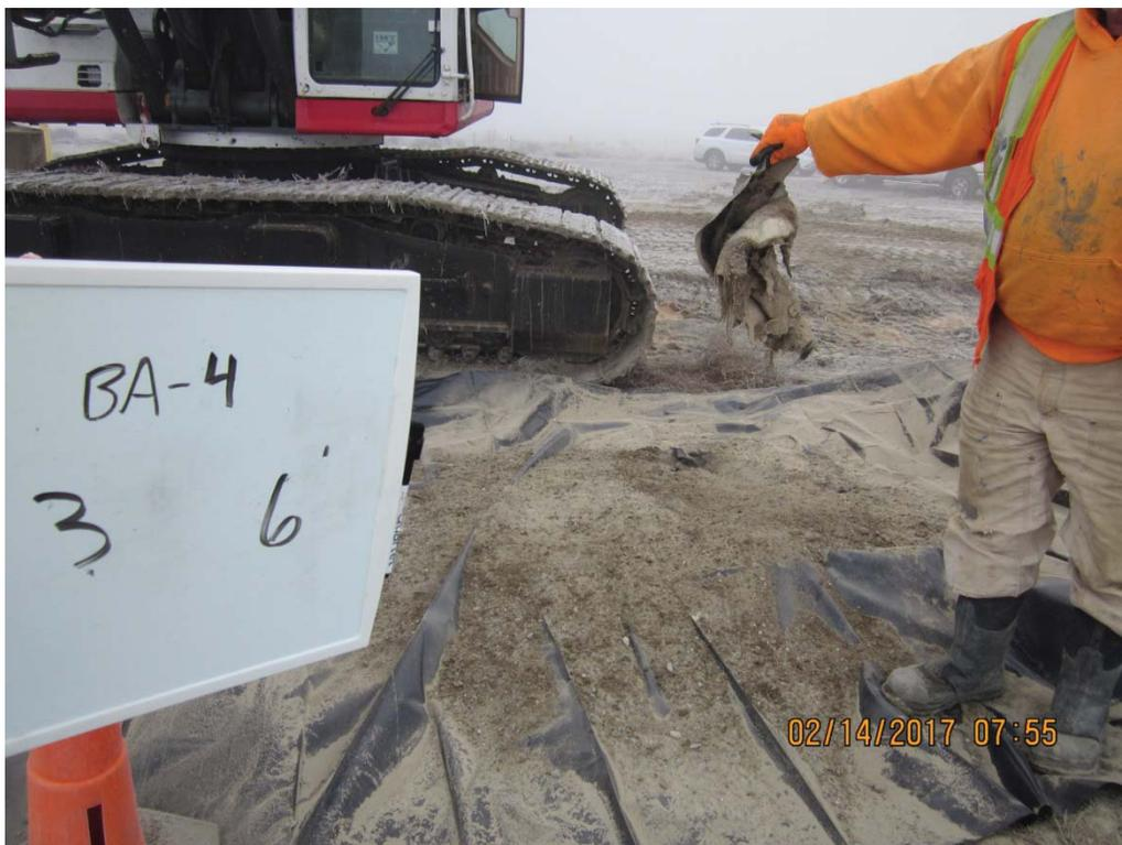
IMG\_5670: Recovery 5 to 6 ft bgs. Piece of Geomembrane recovered. (2/2)
