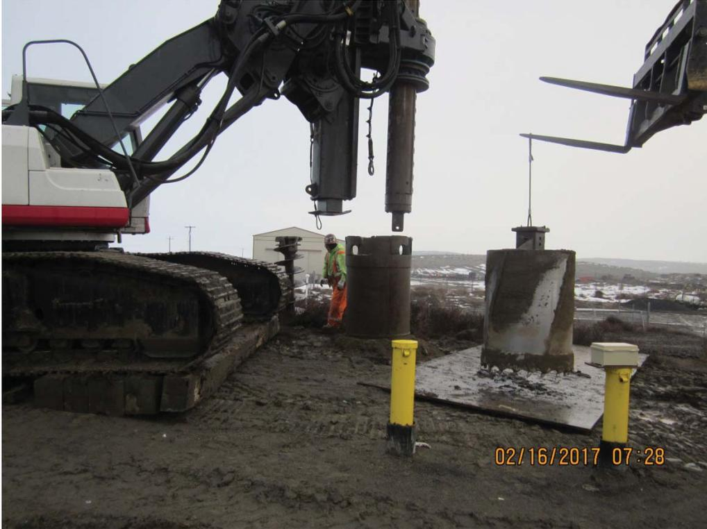
IMG\_5963: Driller setting fall protection casing at surface.
