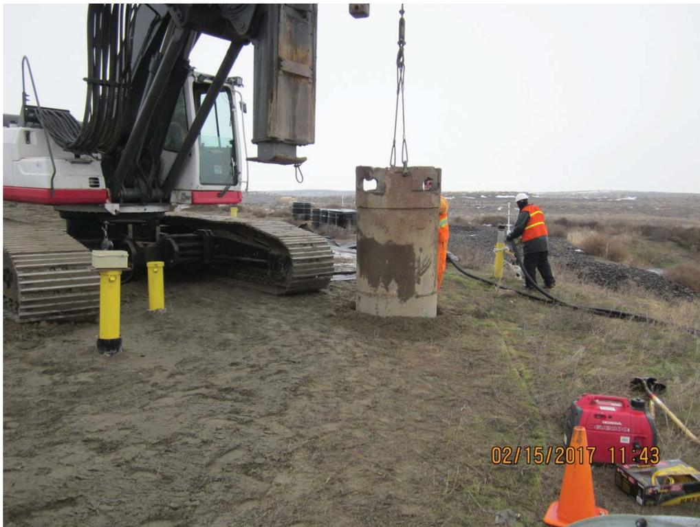
IMG\_5922: Begin drilling and setting fall protection casing at surface. (2/2)
