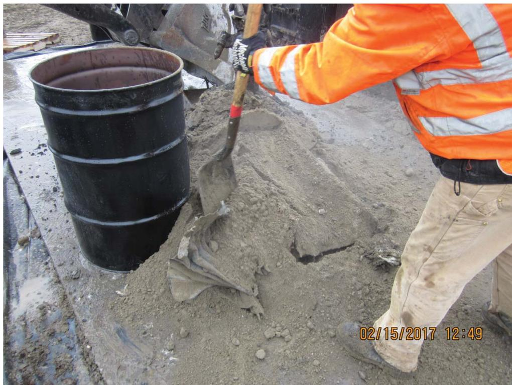
IMG\_5942: Recovery 17 to 18 ft bgs. Piece of Geomembrane recovered. (2/4)
