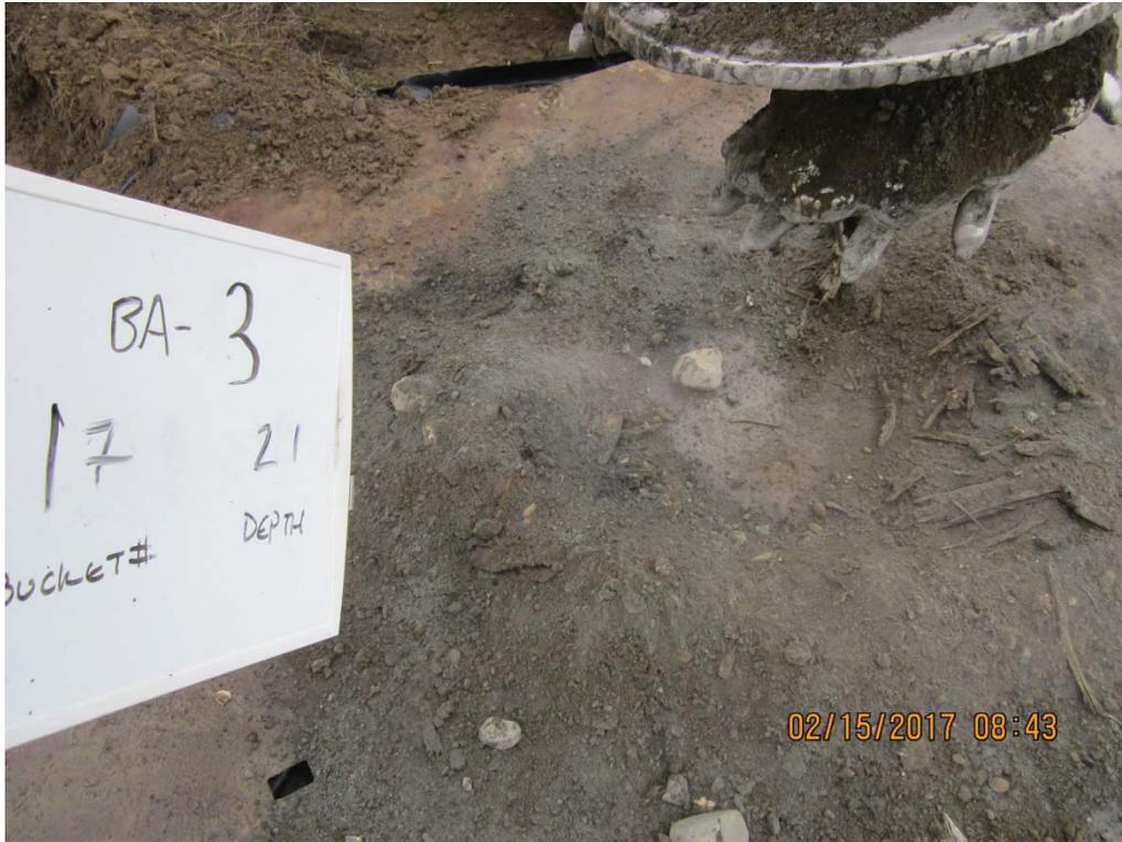
IMG\_5893: Recovery 19.5 to 21 ft bgs. Wood debris recovered on bottom flights of auger. Spread for inspection by Driller's assistant. (2/2)
