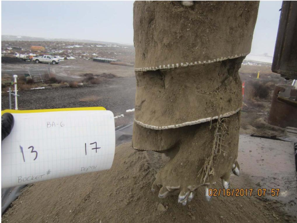
IMG\_5978: Recovery 16 to 17 ft bgs. Piece of Geonet recovered.
