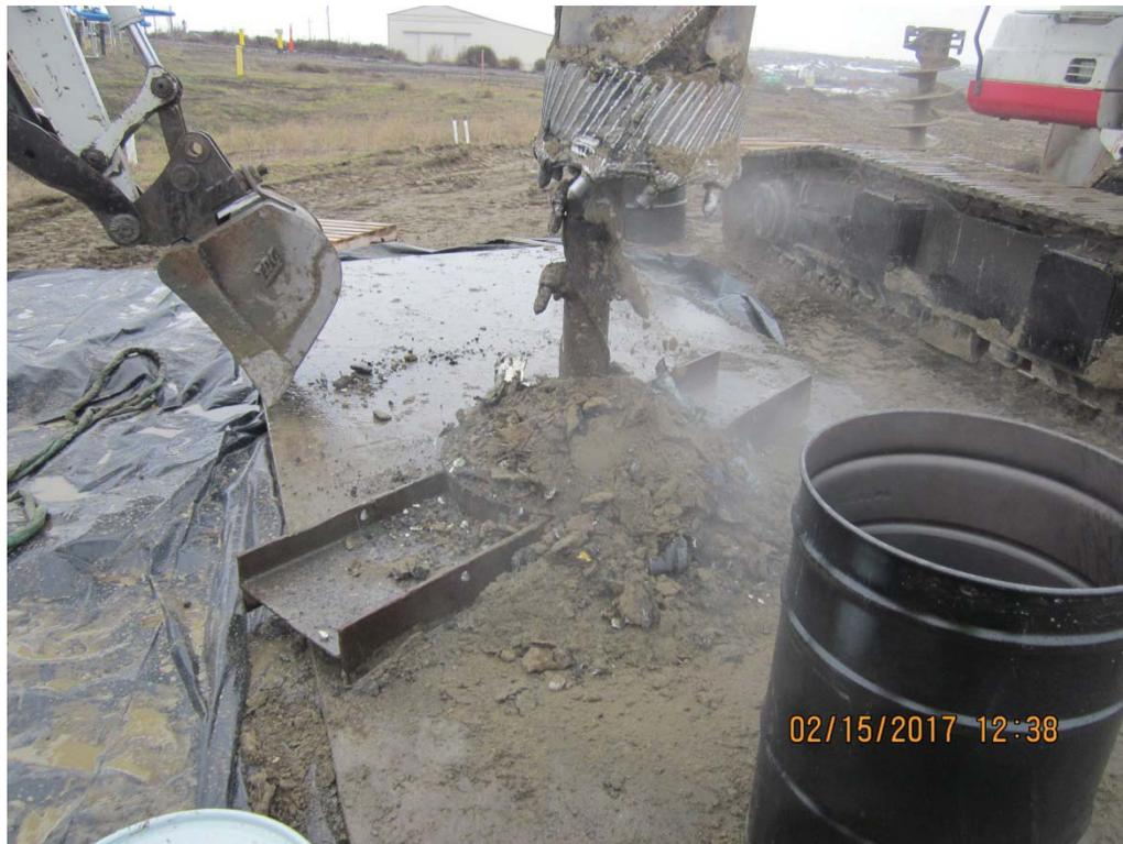
IMG\_5940: Recovery 15 to 17 ft bgs. Driller using roter to dislodge compacted recovered materials from core barrel. (2/2)
