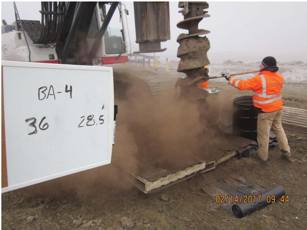
IMG\_5745: Recovery 26 to 28.5 ft bgs. Pass No. 1. (3/15)
