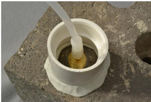
Figure 6. Water dam used for leak detection
