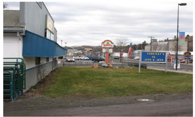
Photograph 8. View looking south across the west side of the Colfax Grange Supply Company building.
