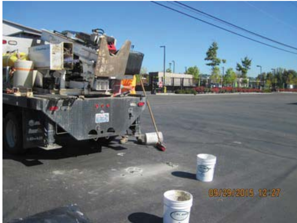
Photograph 1. North side of the KIP parcel facing north-northeast. White powder is bentonite and/or concrete residual from filling temporary soil boring.
