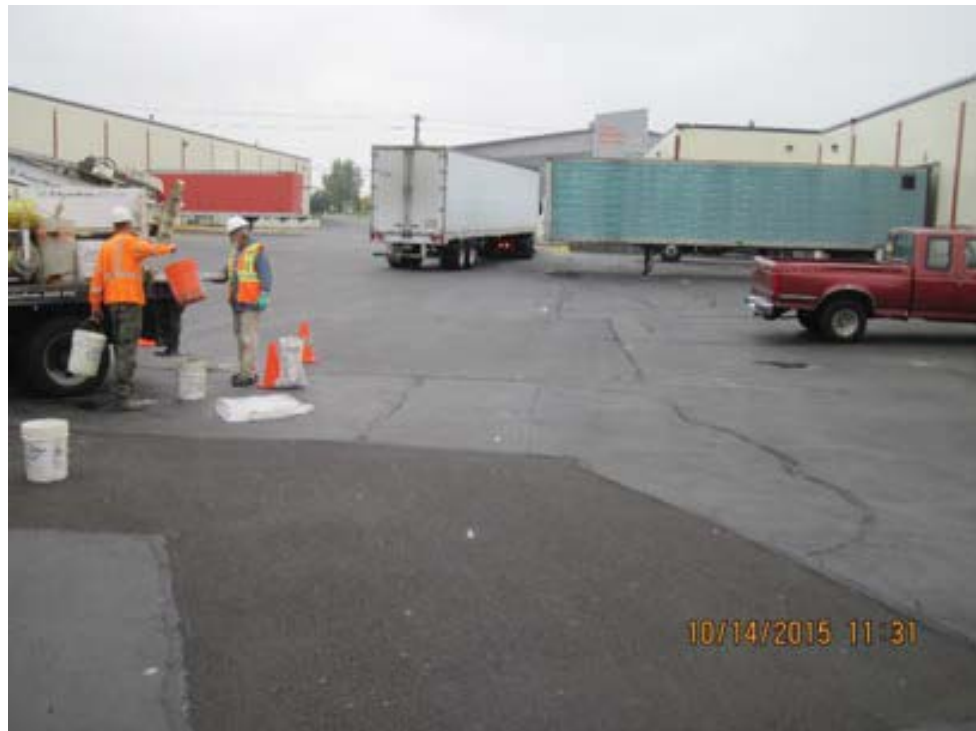
Photograph 4. Central portion of the KIP parcel facing north. Historical pavement patch and sealed crack visible in figure.
