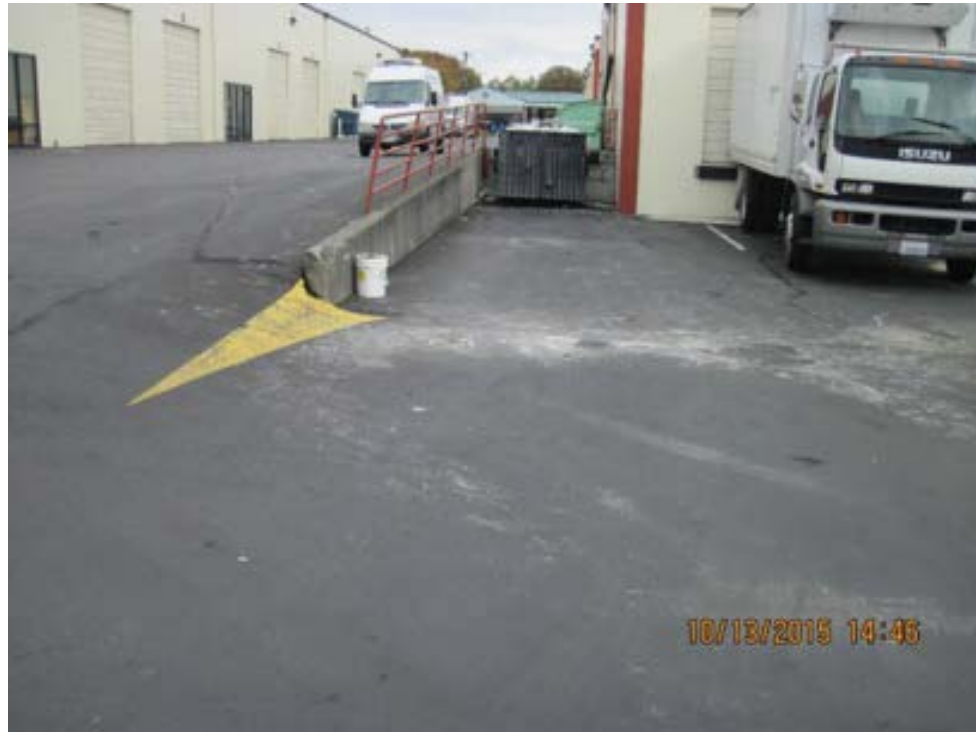
Photograph 3. Central portion of the KIP parcel facing east. White powder is bentonite and/or concrete residual from filling temporary soil boring.
