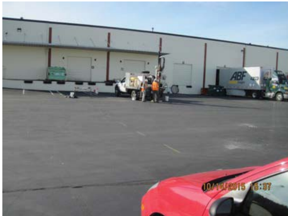
Photograph 5. Central portion of the KIP parcel facing west-northwest. Sealed crack visible in foreground.
