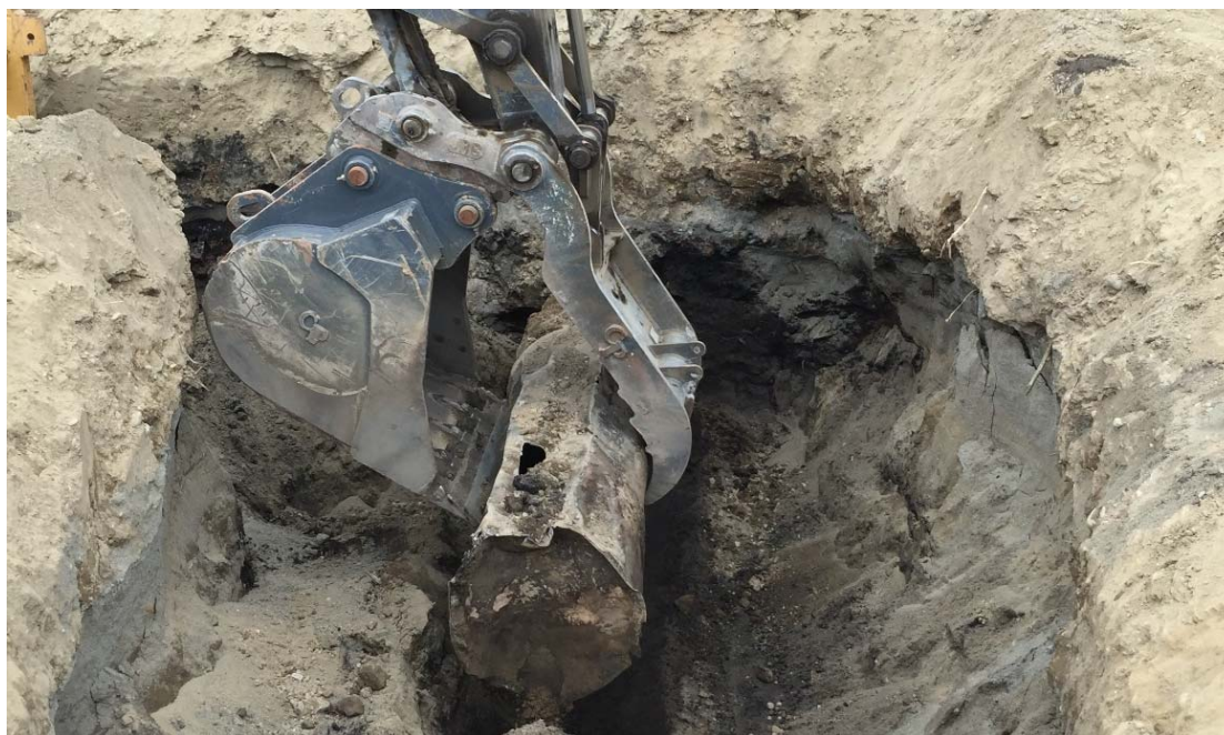
Photograph 15 Close-up of the underground storage tank (UST) after discovery in June 2015.
