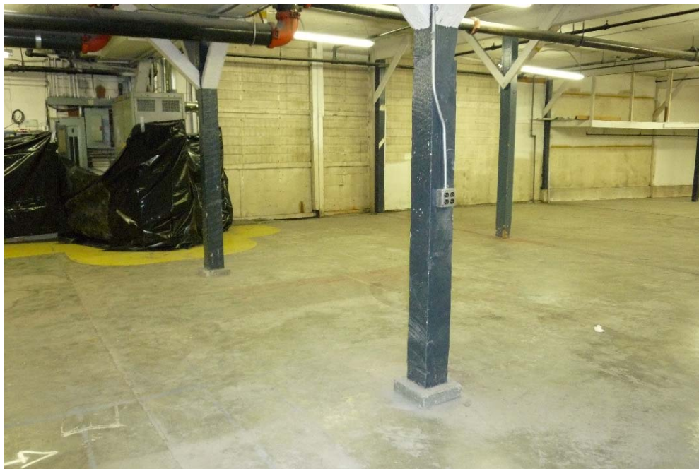
Photograph 2 Scarification of concrete in Building 6 in August 2009.
