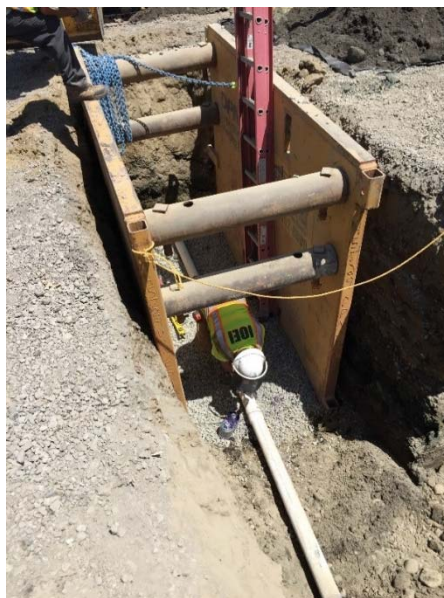
Photograph 17 SVE piping installation in June 2015.
