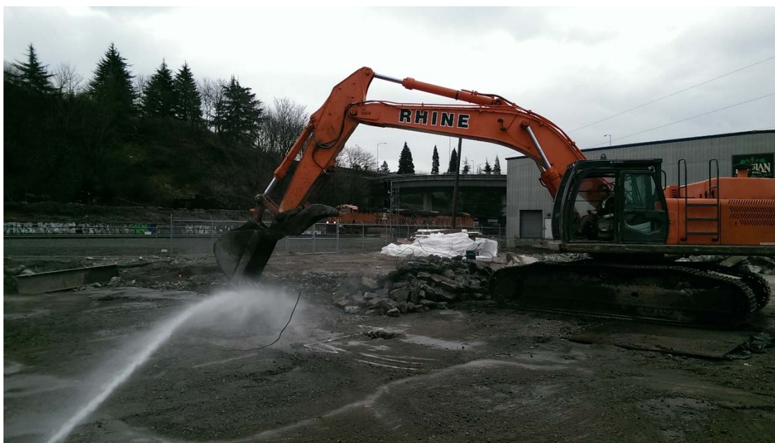
Photograph 5 Concrete slab removal from Building 8 for PCB cleanup in 2015.
