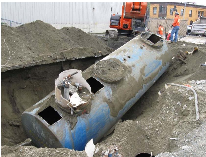
Photograph 3 Top of Tank 3 during removal (example of product tank) in 2010.
