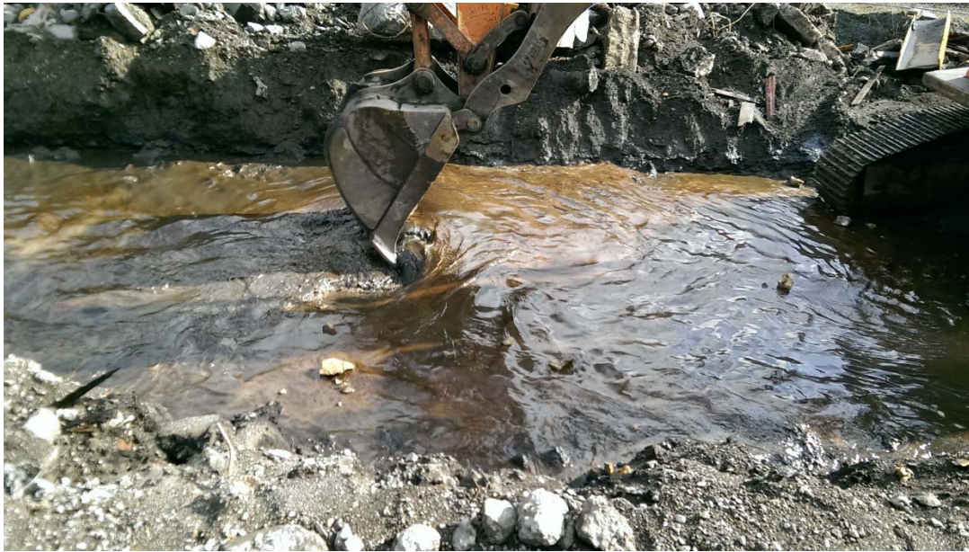
Photograph 11 Oxidant mixing in piping excavation phase 1 in March 2015.
