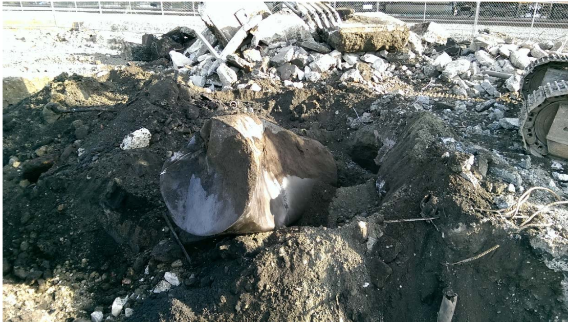
Photograph 12 UST after discovery on March 5, 2015. View is to the east.
