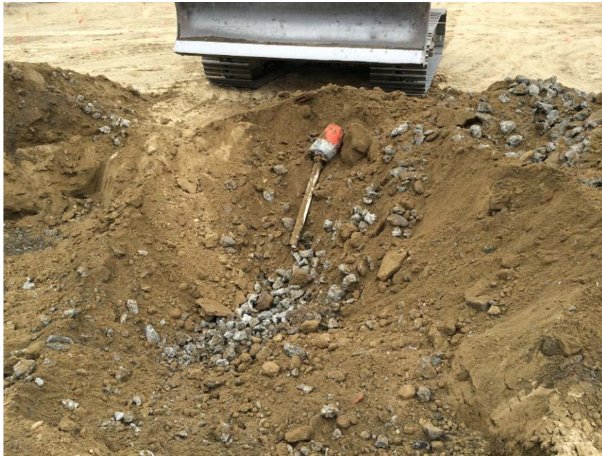
Photograph 13 KM-03 well abandonment in June 2015.
