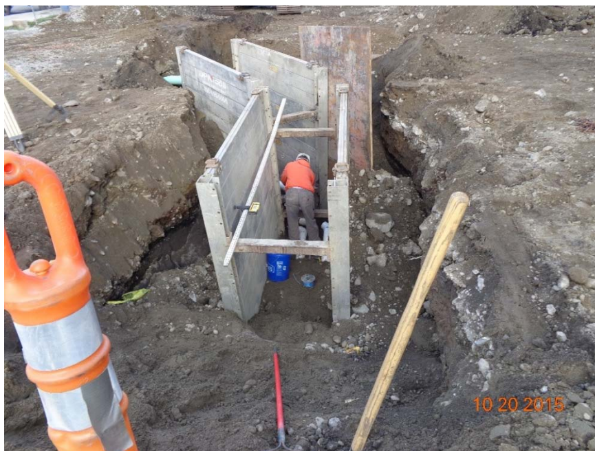
Photograph 19 Installation of the SVE piping in October 2015.
