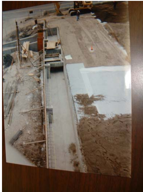
Photograph 1 Vapor Barrier Installation of the south building.
