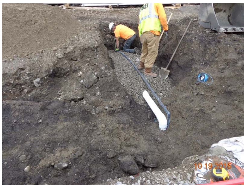
Photograph 18 Installation of the SVE piping in October 2015.
