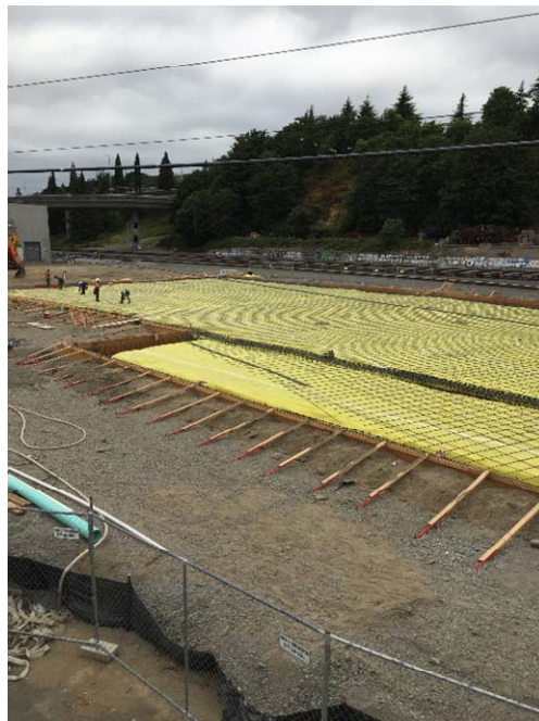
Photograph 14 Vapor barrier installation in June 2015.
