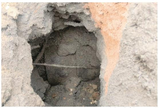
Photograph 2. The 8-inch-diameter concrete inlet pipe outside (west) of the junction box curving west to southwest via conjoined bell joints (September 5, 2017).
