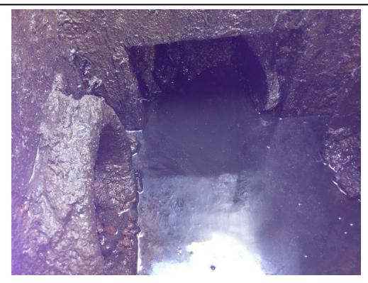
Photograph 5. View of the 8-inch-diameter concrete pipe on the north side of the junction box. A buildup of rock and mud was visible inside all three pipes (September 22, 2017).
