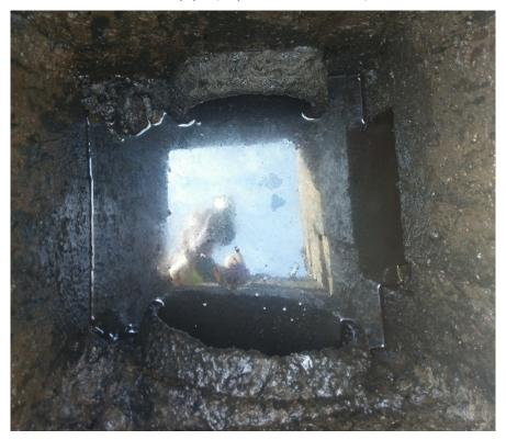
Photograph 4. Inside view of the junction box. The box interior includes the 12-inch-diameter concrete outlet pipe to Outfall LLO-07 (bottom), the 8-inch-diameter concrete inlet pipe traveling north from the box toward the barrier wall and asphalt cap (right), and the 8-inch-diameter concrete inlet pipe traveling west toward the property line (top) (September 22, 2017).
