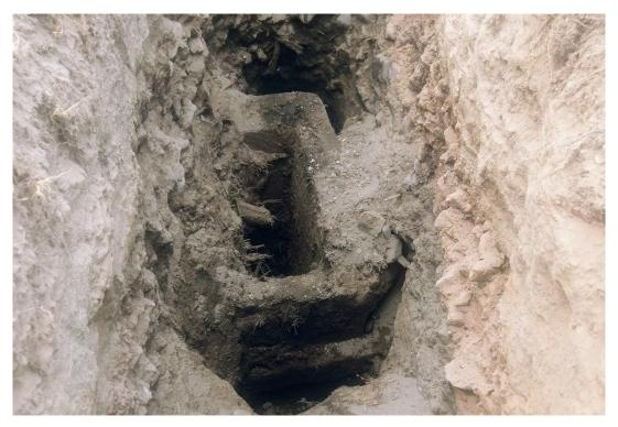
Photograph 1. The wooden junction box viewed looking northwest, in line with the 12-inch-diameter concrete outlet pipe (September 5, 2017).
