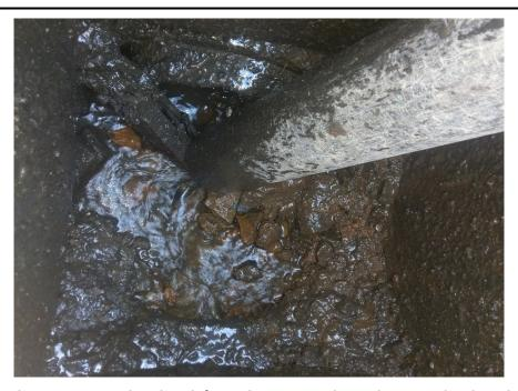
Photograph 3. Clearing out mud and rock from the junction box. Photograph taken during ebb tide, causing water (river water) to flow into the box from the inlet pipes and out of the box through the outlet pipe (September 22, 2017).
