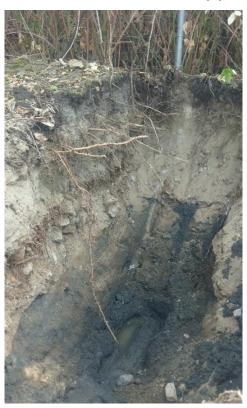
Photograph 6. View of the exposed 8-inch-diameter pipe on the west side of the junction box at the property line (September 22, 2017)
