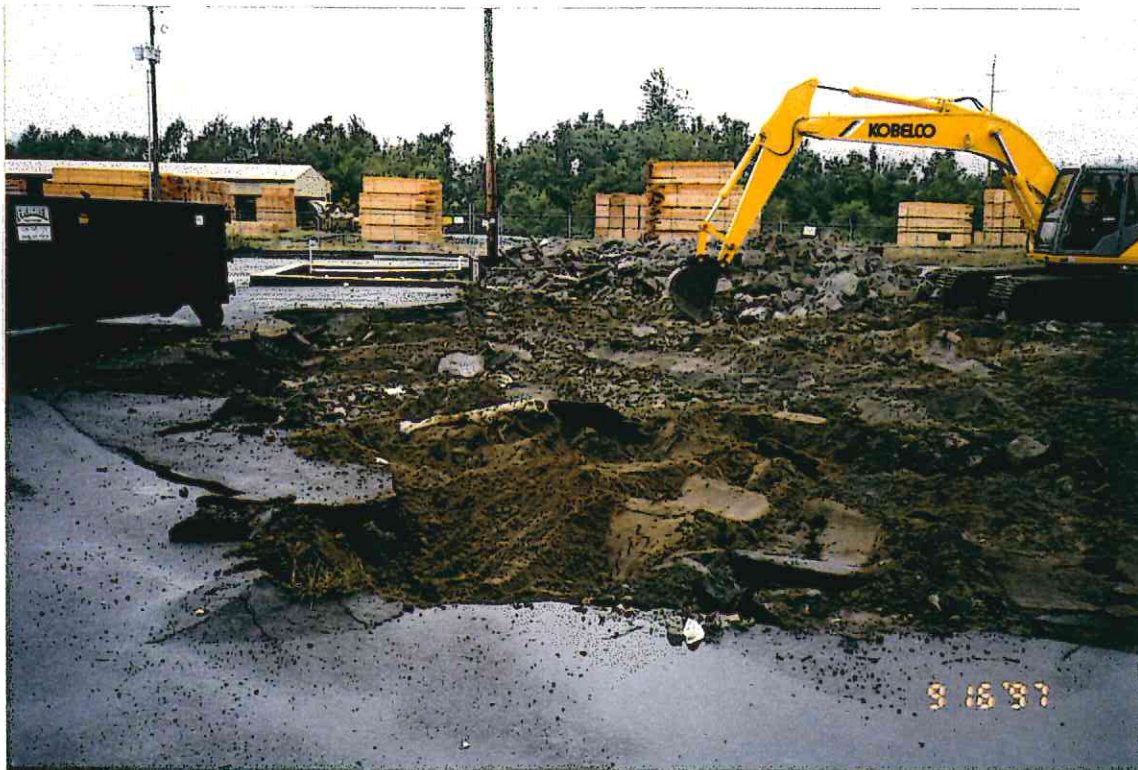
5. Track-hoe breaking up concrete in former tank farm.
