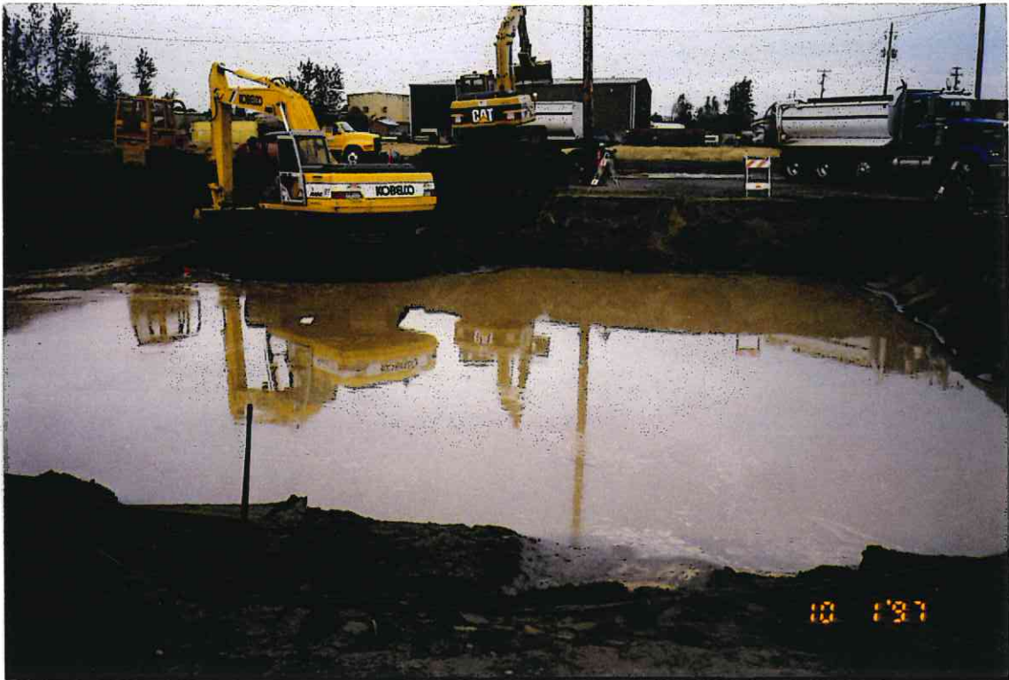
19. Excavation to 6 feet below ground surface.
