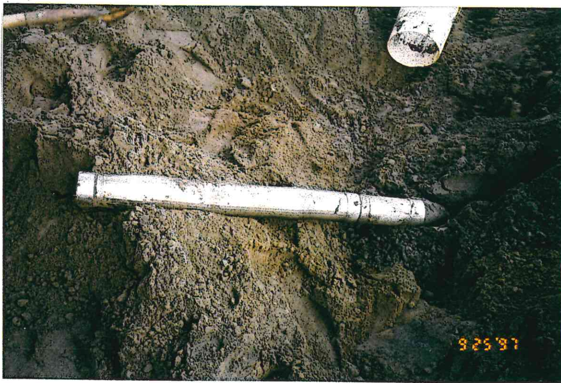
14. MC-R pulled from ground and bucket from dry well in background.
