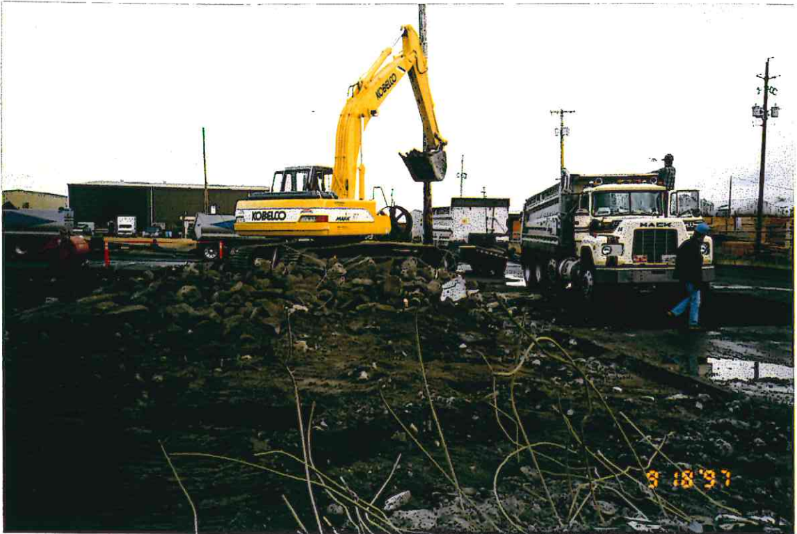
7. Loading concrete onto trucks for disposal at Rabanco Landfill.
