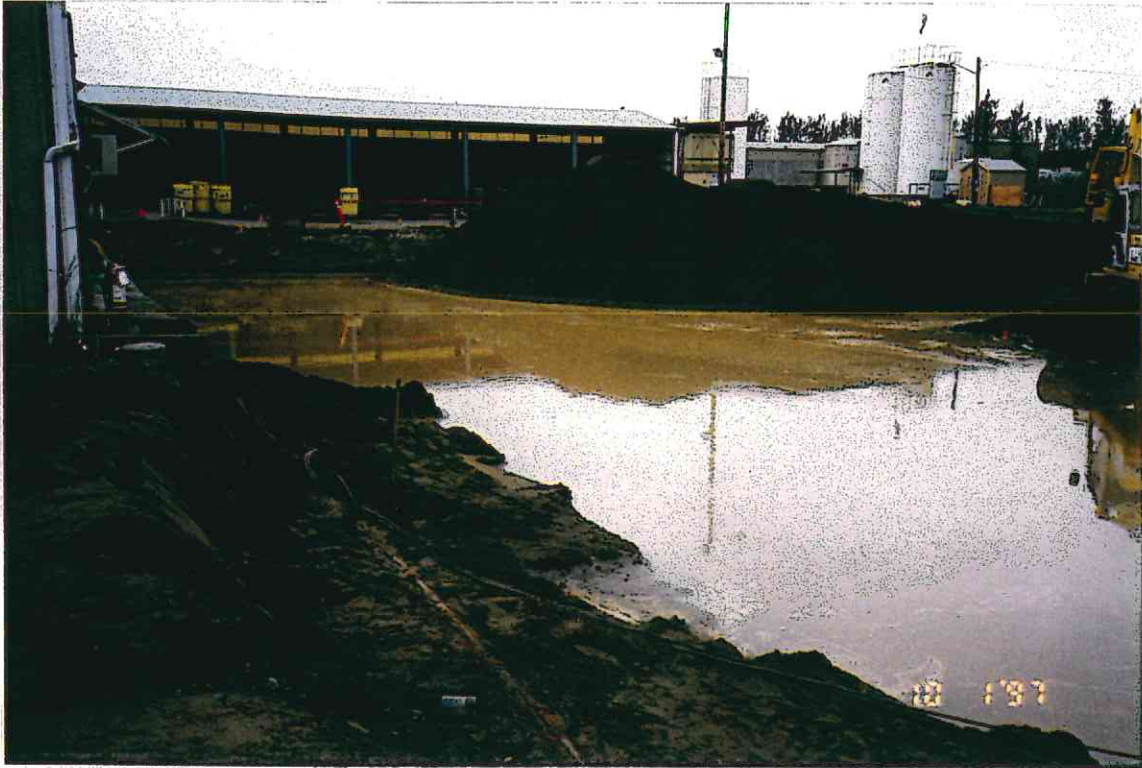
17. Excavation filled with water from approximately 4 feet below ground surface.
