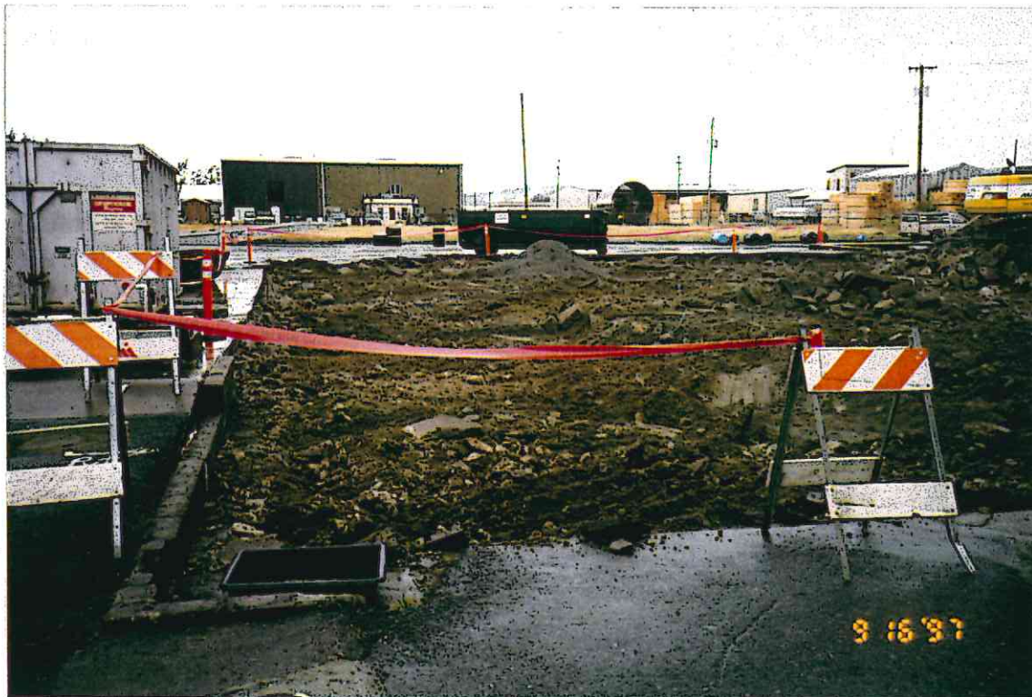
6. All concrete broken up and hauled to Rabanco Landfill.
