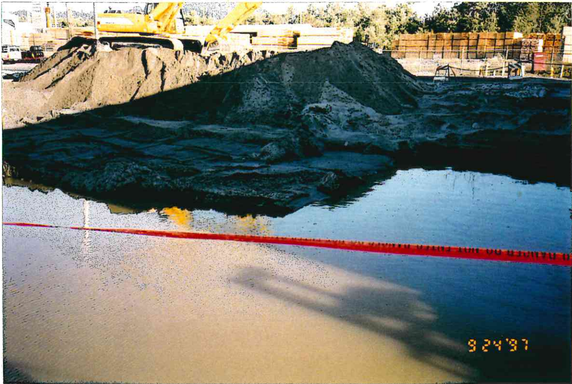
11. Soil excavated to 6 feet below ground surface.
