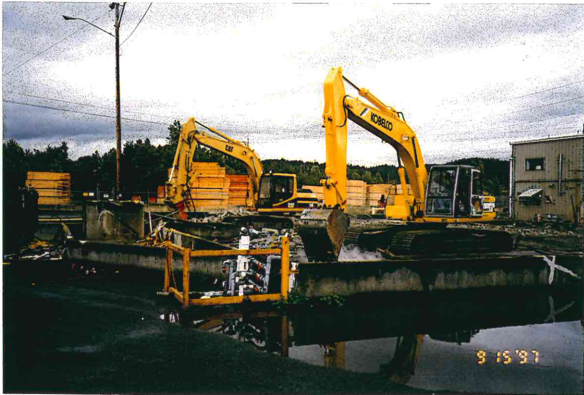
3. Track-hoe breaking up concrete in former tank farm.
