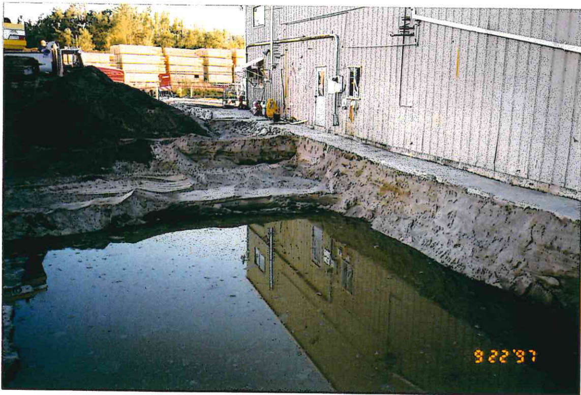
10. Soil excavated to approximately 3-4 feet below ground surface.
