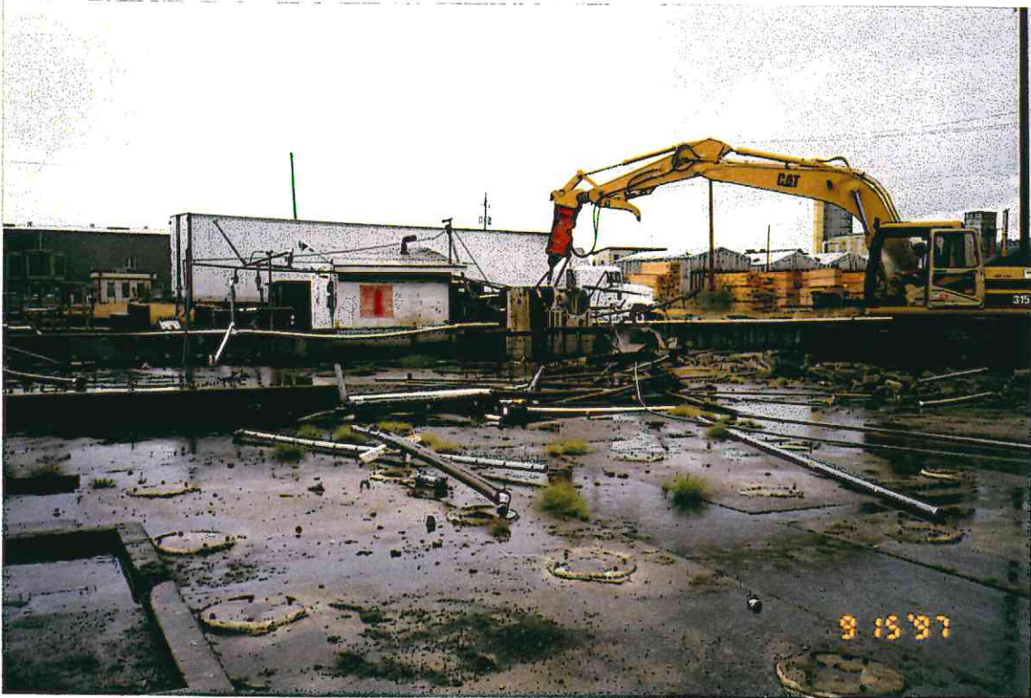
1. Track-hoe demolishing the remainder of above-ground piping from the former tank farm.
