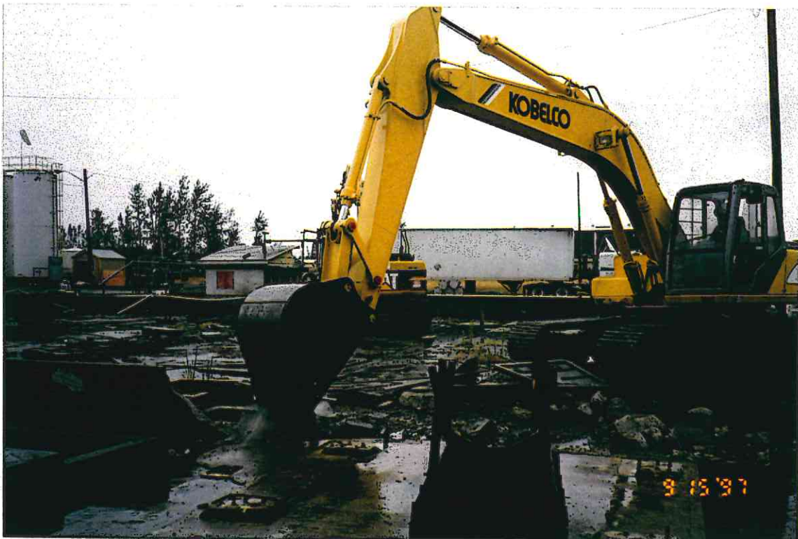
4. Track-hoe breaking up concrete in former tank farm.
