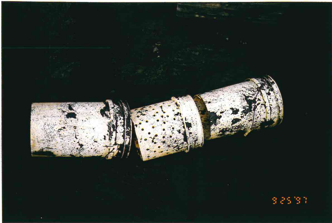
15. Dry well pieced together on ground surface for inspection. Notice the bottoms of the 5-gallon buckets are cut out and drain holes were drilled into the middle bucket.
