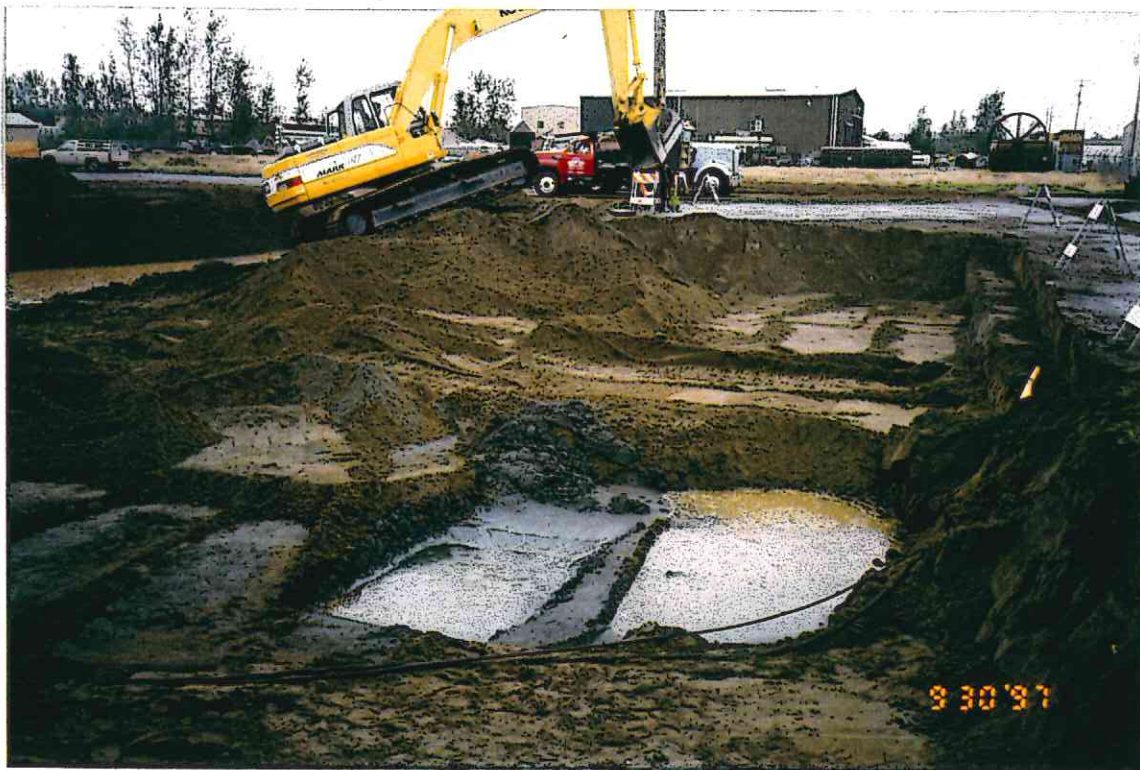
16. Continue excavation to 6 feet below ground surface across the tank farm.
