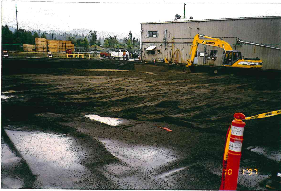
21. Fill in excavation with pre-load.
