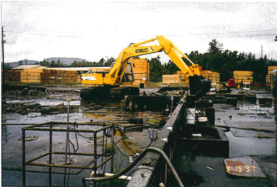
1. Track-hoe demolishing the remainder of above-ground piping from the former tank farm.
