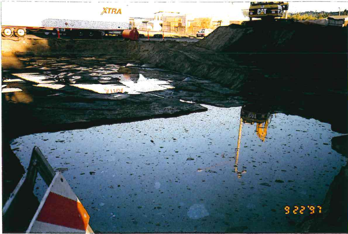
9. Soil excavated to approximately 3-4 feet below ground surface.
