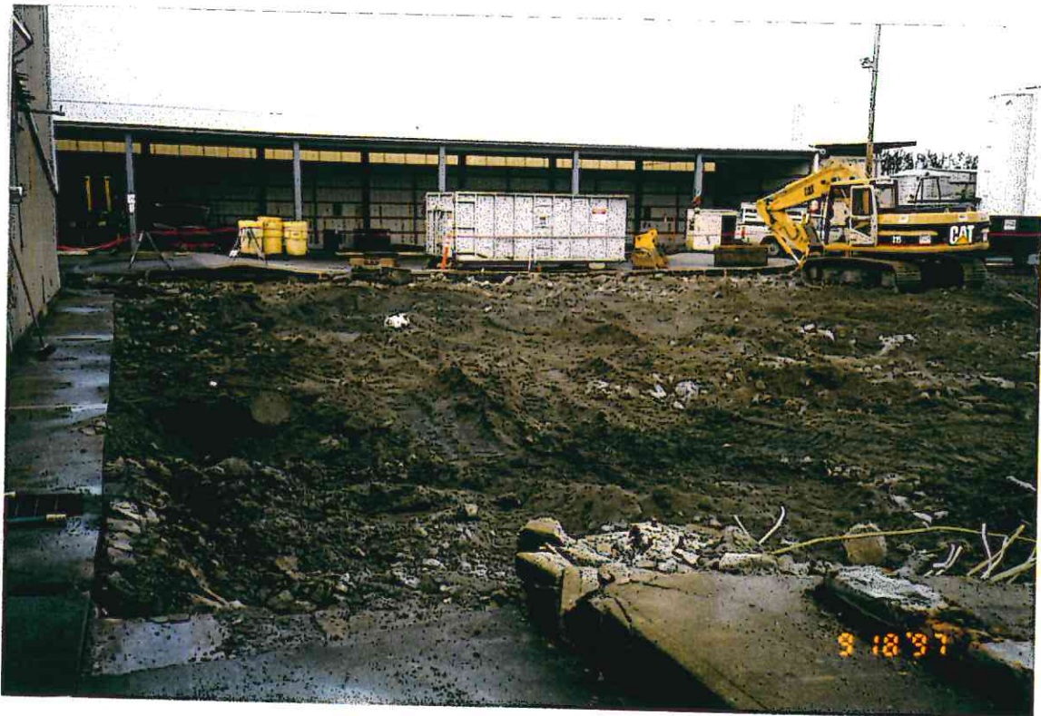
8. Beginning of soil removal.
