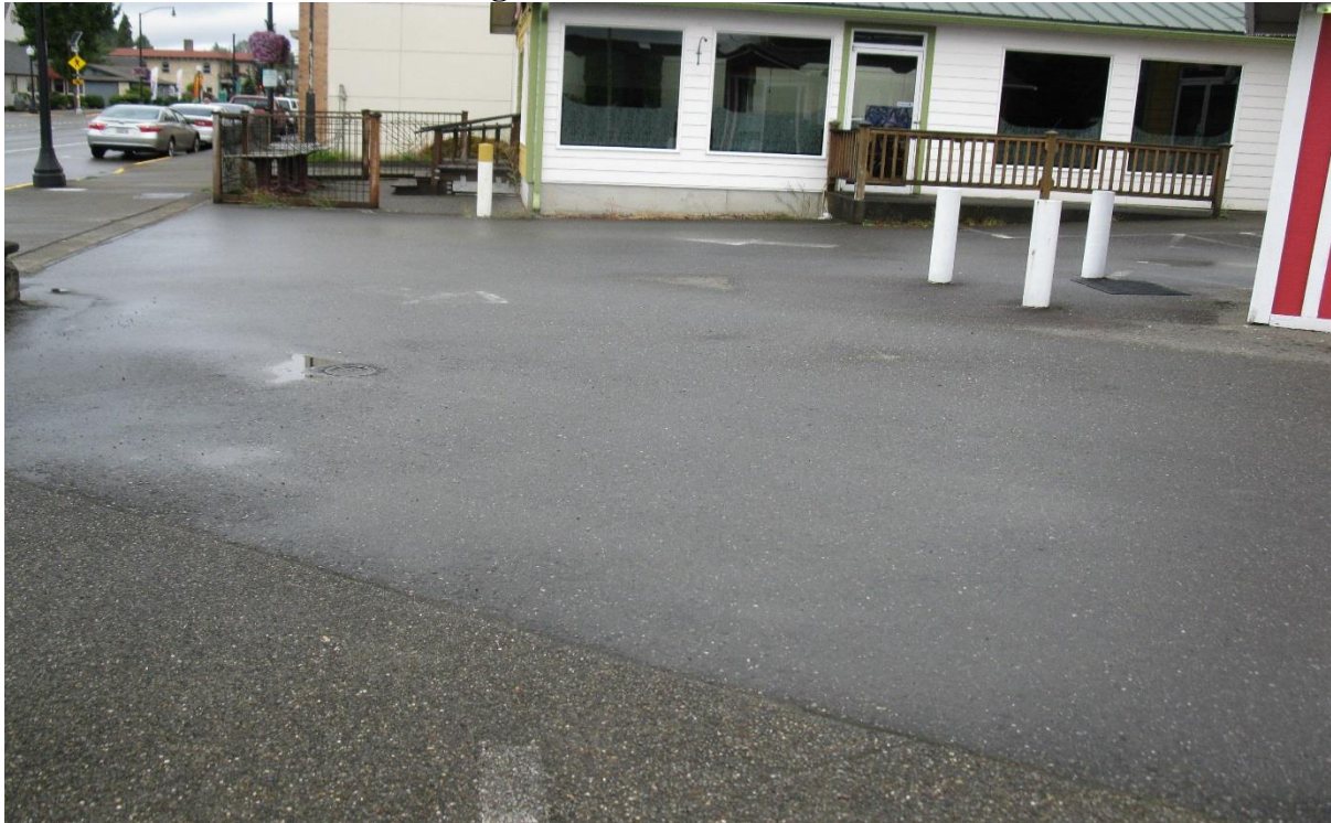
Photo 3: Approximate Area of Soil Contamination Left-in-Place and Asphalt Cap and Groundwater Monitoring Well – from the East
