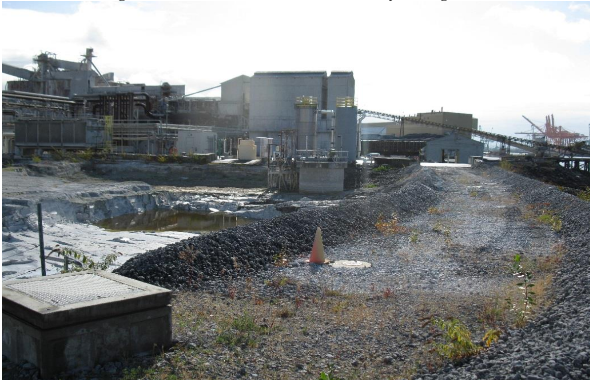
Photo 6: Monitoring Well at Waterfront North of Secondary Setting Pond–from the North
