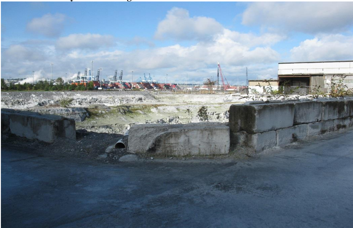
Photo 4: Secondary Lime Settling Pond – from the Southwest
