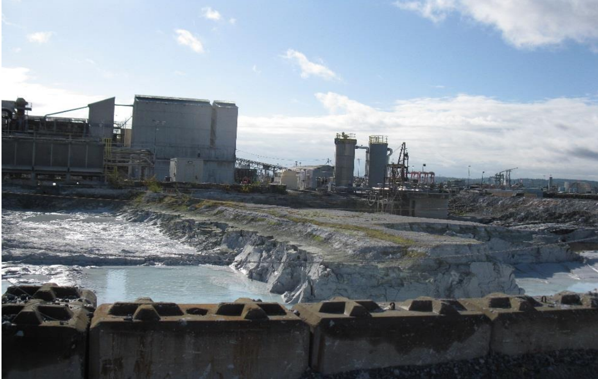
Photo 7: Secondary Settling Pond – from the North
