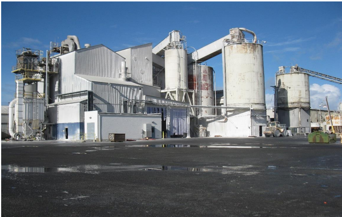
Photo 1: Main Plant – from the East
