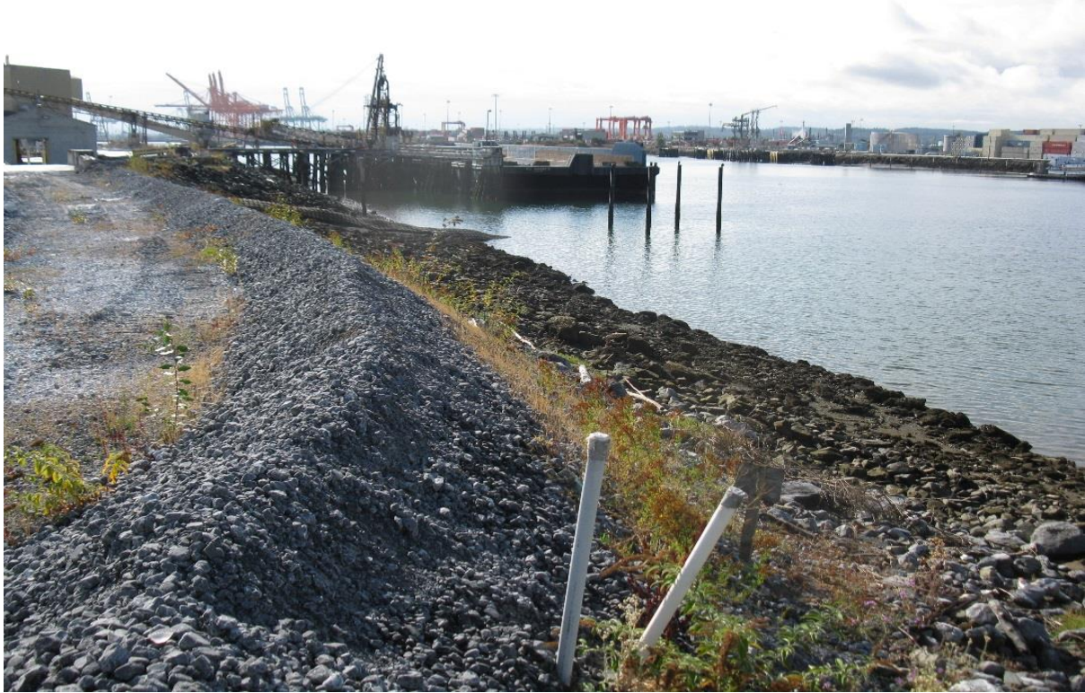
Photo 5: Blair Waterway South of the Secondary Settling Pond – from the North
