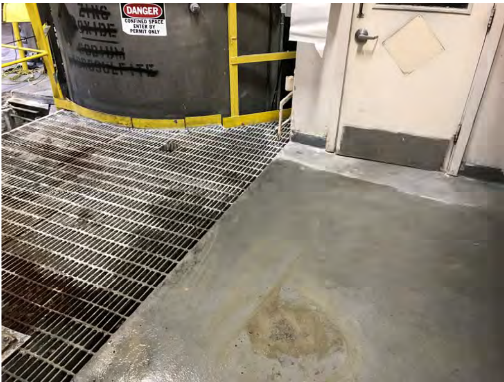
Photograph 6: SB21 adjacent to subgrade tank vault in Make Tank Room
