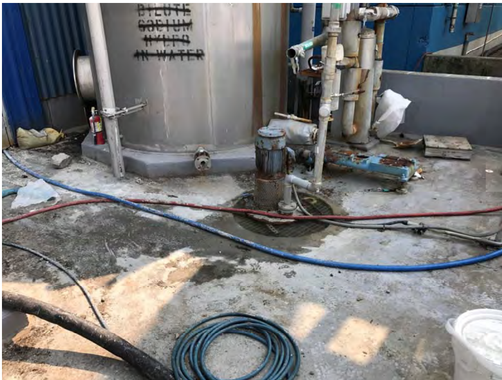
Photograph 10: Sump outside Zinc Oxide Dryer Room (SB20)
