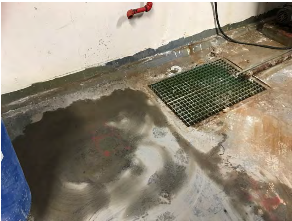
Photograph 8: Sump in Formulation Room (SB23)
