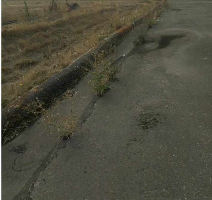
Photograph 5. Crack in the asphalt with growing vegetation along the south edge of the cap (looking west).
