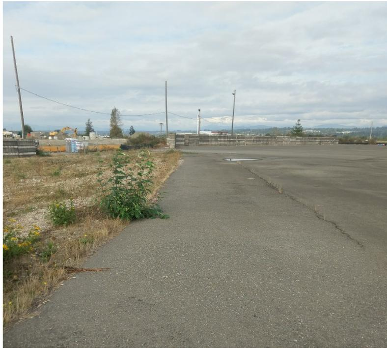
Photograph 1. Crack in asphalt on northwest side of the cap (looking north).
