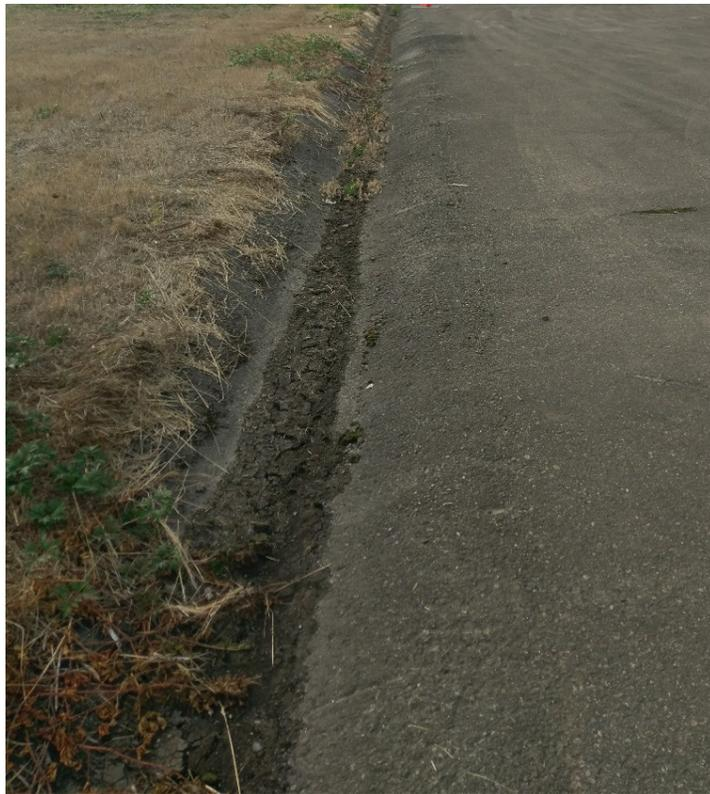
Photograph 6. Accumulated sediment within the drainage ditch along the south edge of the cap (looking west).
