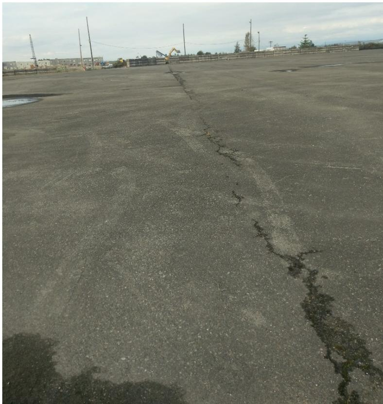
Photograph 2. Crack in asphalt through the center of the cap (looking north).
