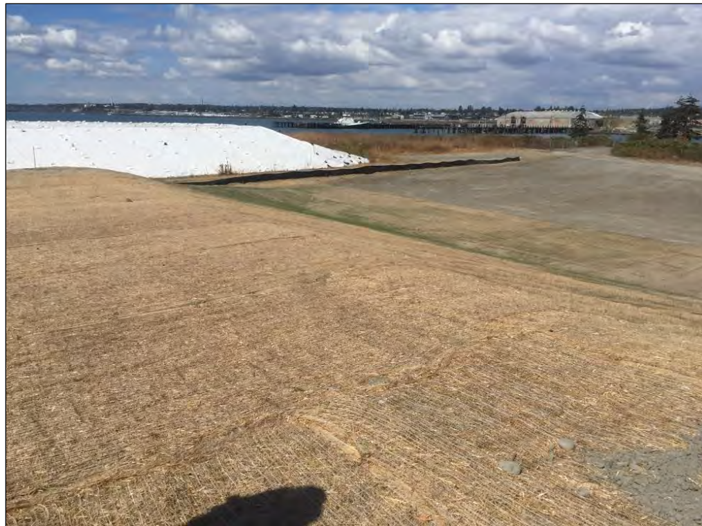
6. Top of pile looking northwest, silt fence visible, some grass visible on northern slope. Per survey, fill needs to be added to areas north of pile to facilitate drainage.
