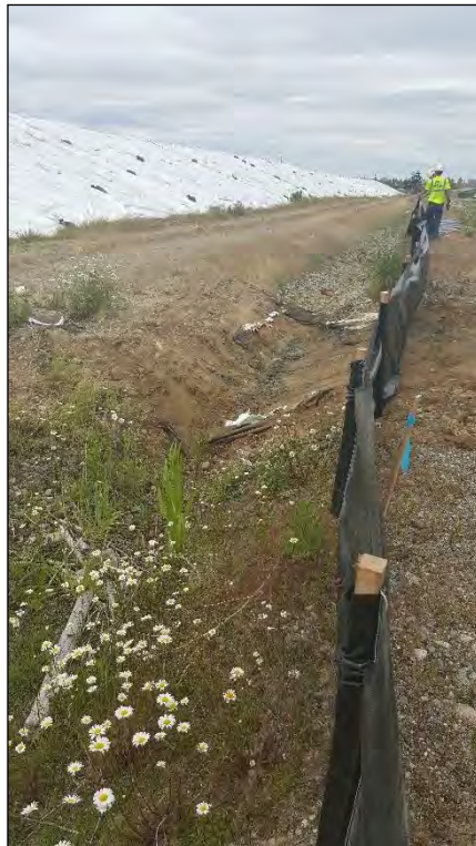
7. Ditches have been connected for stormwater flow. A culvert was installed here after this photo was taken.
