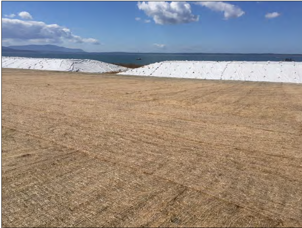
37. Looking west from top of northern stockpile.
