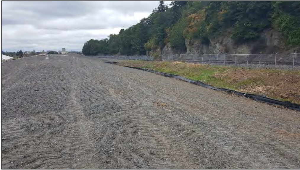
25. Looking north toward northern stockpile from middle of south stockpile. Erosion control matting being placed.
