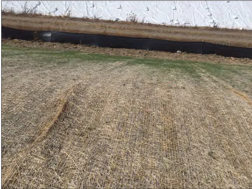
32. Looking down the west side of the northern stockpile
