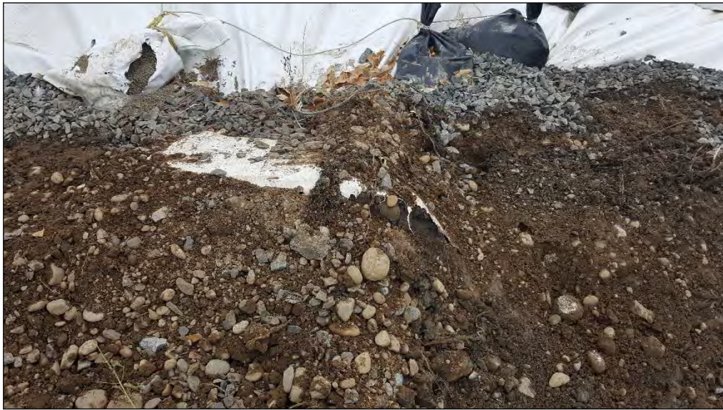
26. Repairs made to damaged stockpile cover.
