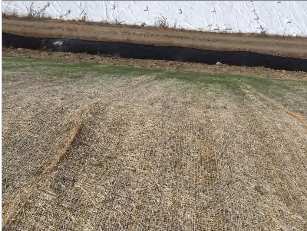
5. Top of pile looking west, down the western slope, silt fence visible, grass visible.
