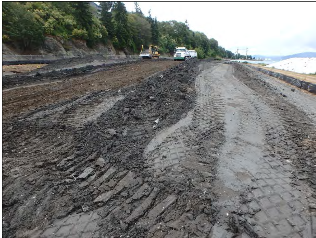
20. Construction of southern stockpile.
