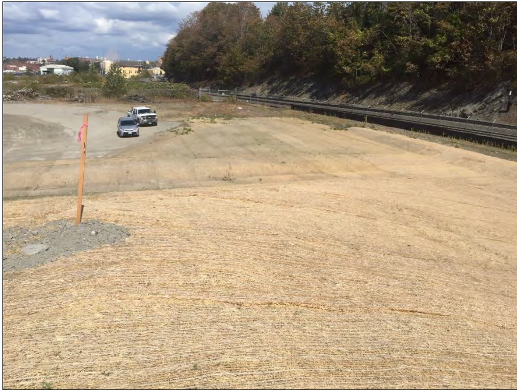
33. Looking north from top of northern stockpile.
