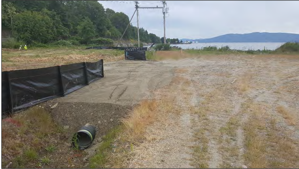
6. Culvert installed at location of approach ramp to stockpile.
