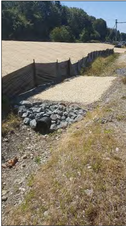
29. Previously incomplete culvert has been completed.
