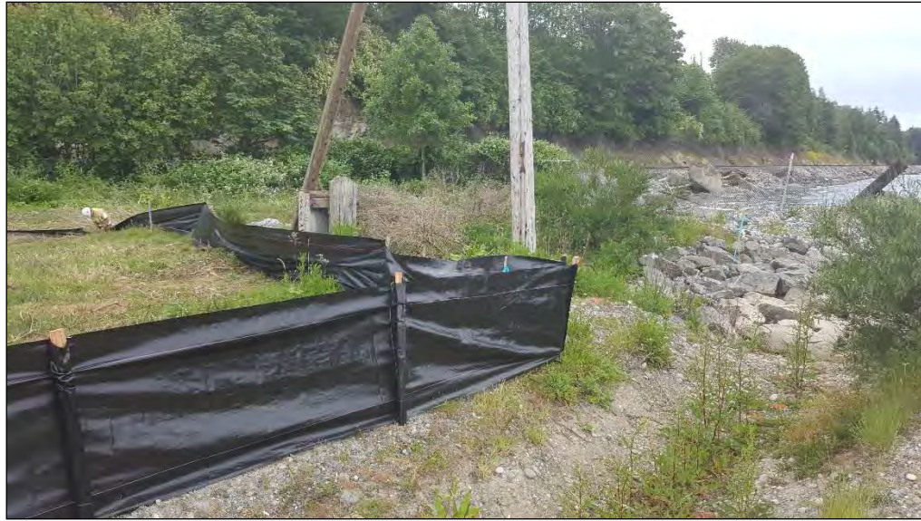
10. Silt fence installed north of planned area to avoid existing structures.
