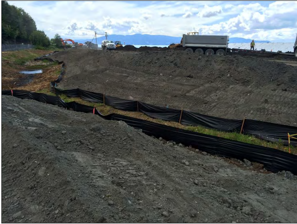
21. Looking south from top of north stockpile.
