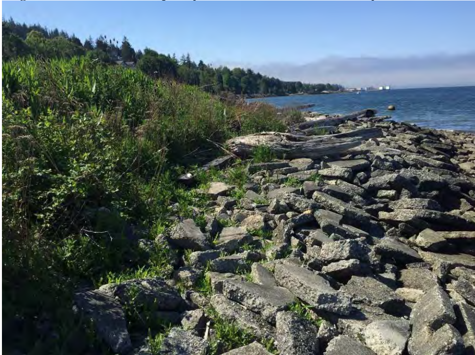
Photograph 4. Weedy grasses and forbs and extensive coverage of angular concrete between the upland and the MHHW in the southern portion of the Site.
