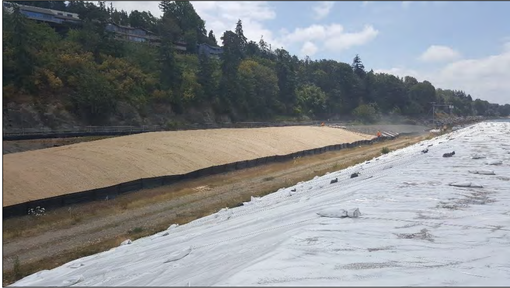
23. Erosion control matting being installed on southern stockpile.
