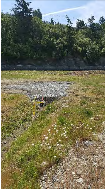
5. Temporary culvert installed between the two stockpiles.
