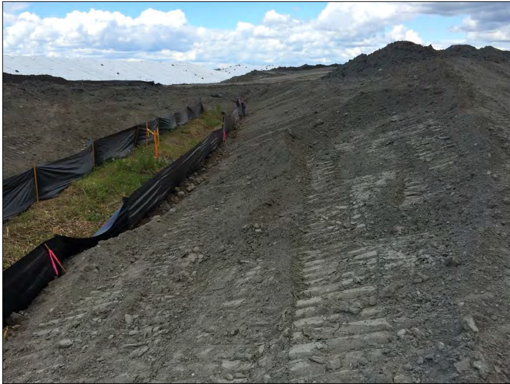
22. Looking west between the two stockpiles. Note silt fence has been repaired.
