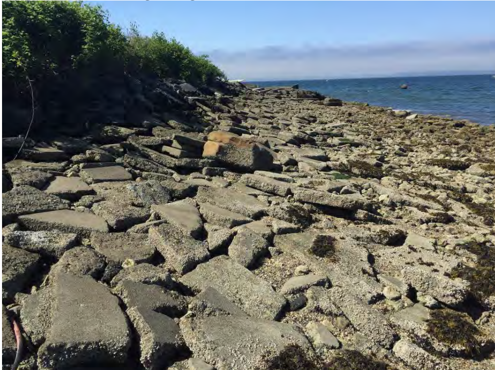
Photograph 8. Extensive coverage of angular concrete below the MHHW within the middle of the Site.
