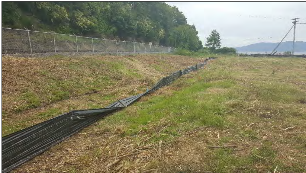
9. Silt fence installed around perimeter of stockpile areas.
