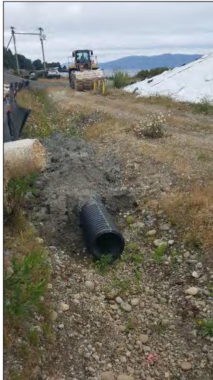
24. Incomplete culvert. Looking to the south.
