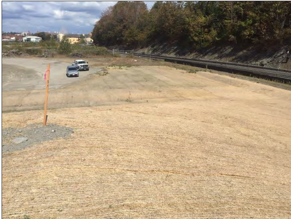
3. Top of pile looking north. Rail tracks on right
