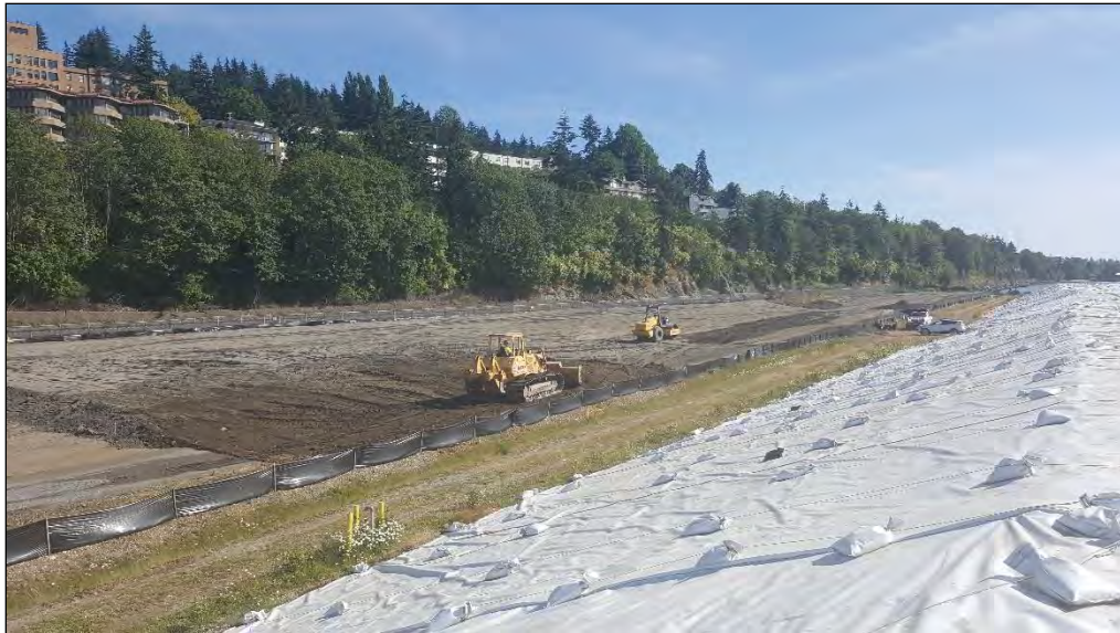
13. Looking south from top of north existing stockpile.
